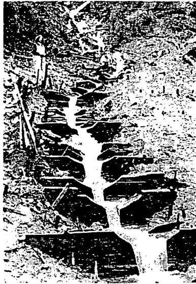
FIGURE 7. Redwood slat check dams were installed in a newly excavated stream channel to prevent downcutting of the stream bed and to help stabilise stream banks. They convey winter flows through broad, high-flow spillways. Each dam is ponding water, and sediment will settle out in the basin up to the height of the spillway. Note the close spacing of check dams, and the rock energy dissipation below the spillways. Stem cuttings of willow are planted on both banks to accelerate revegetation.
