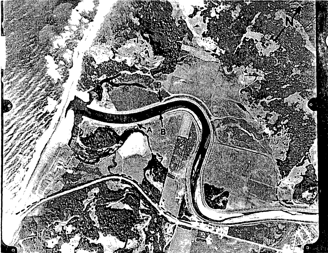
Figure 3. Redwood Creek showing the points of proposed options for restoration: levee spillway, (A); partial levee removal, (B); levee relocation, (Dashed line).
