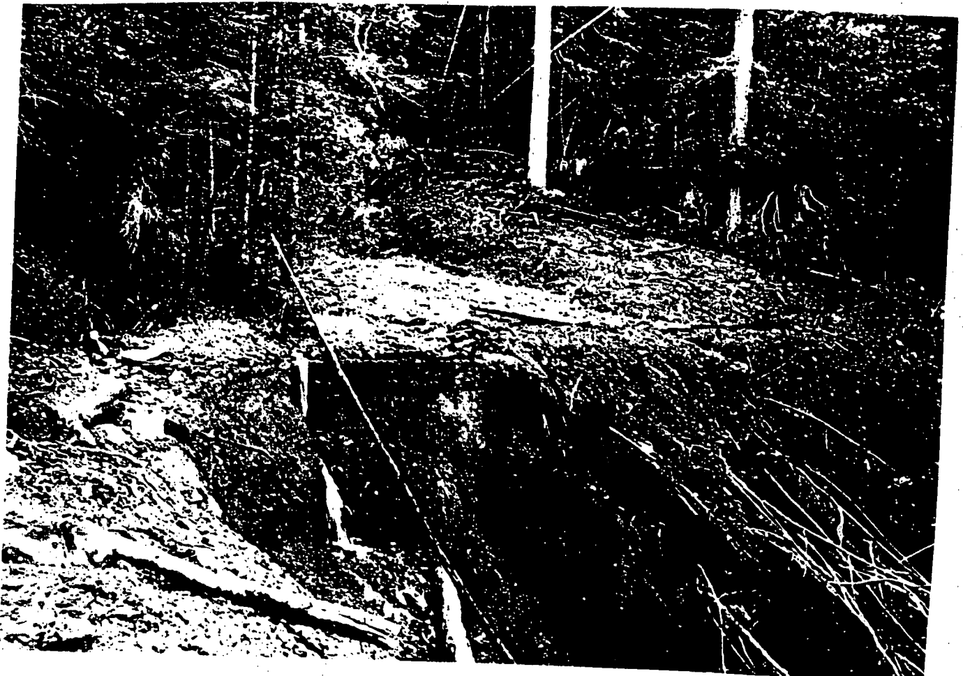
Photo #8: Stream Crossing Failure- This road stream crossing is on Road 15N75 in the Elk Creek Watershed (Doolittle tributary), Happy Camp Ranger District. Failure of the fill was caused by a debris flow which originated by a small fill failure on the same road where it crossed the head of the debris flow channel. Photo summer of 1997 by J.d.I.F.
