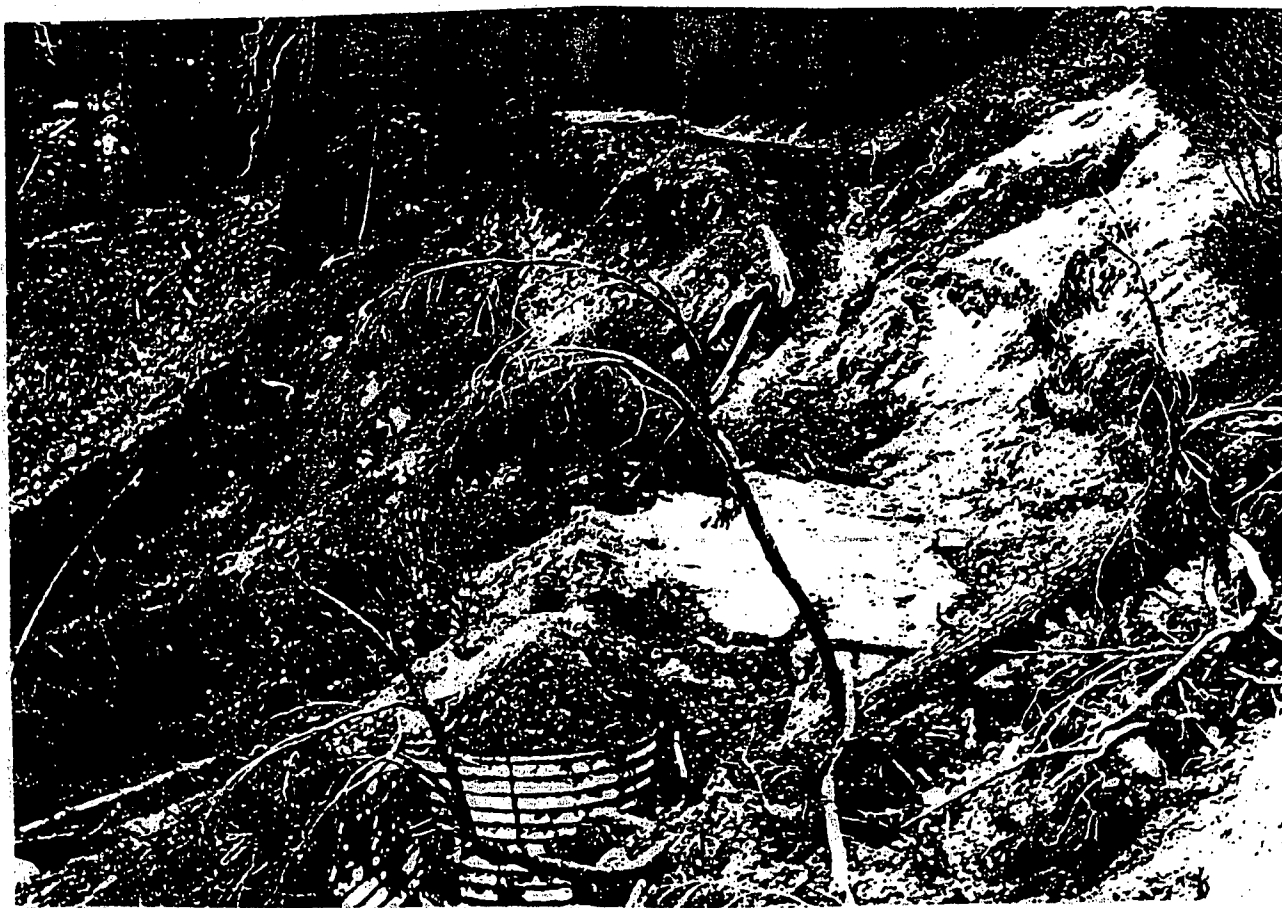
Photo #5: Fill Failure- This fill failure is on Road 44N45 in the Canyon Creek Watershed, Scott River Ranger District. Failure was a result of fill saturation with some additional water contributed to the site by the inside road ditch. Photograph by Ed Rose, spring, 1997. This site was subsequently repaired with a retaining wall.
