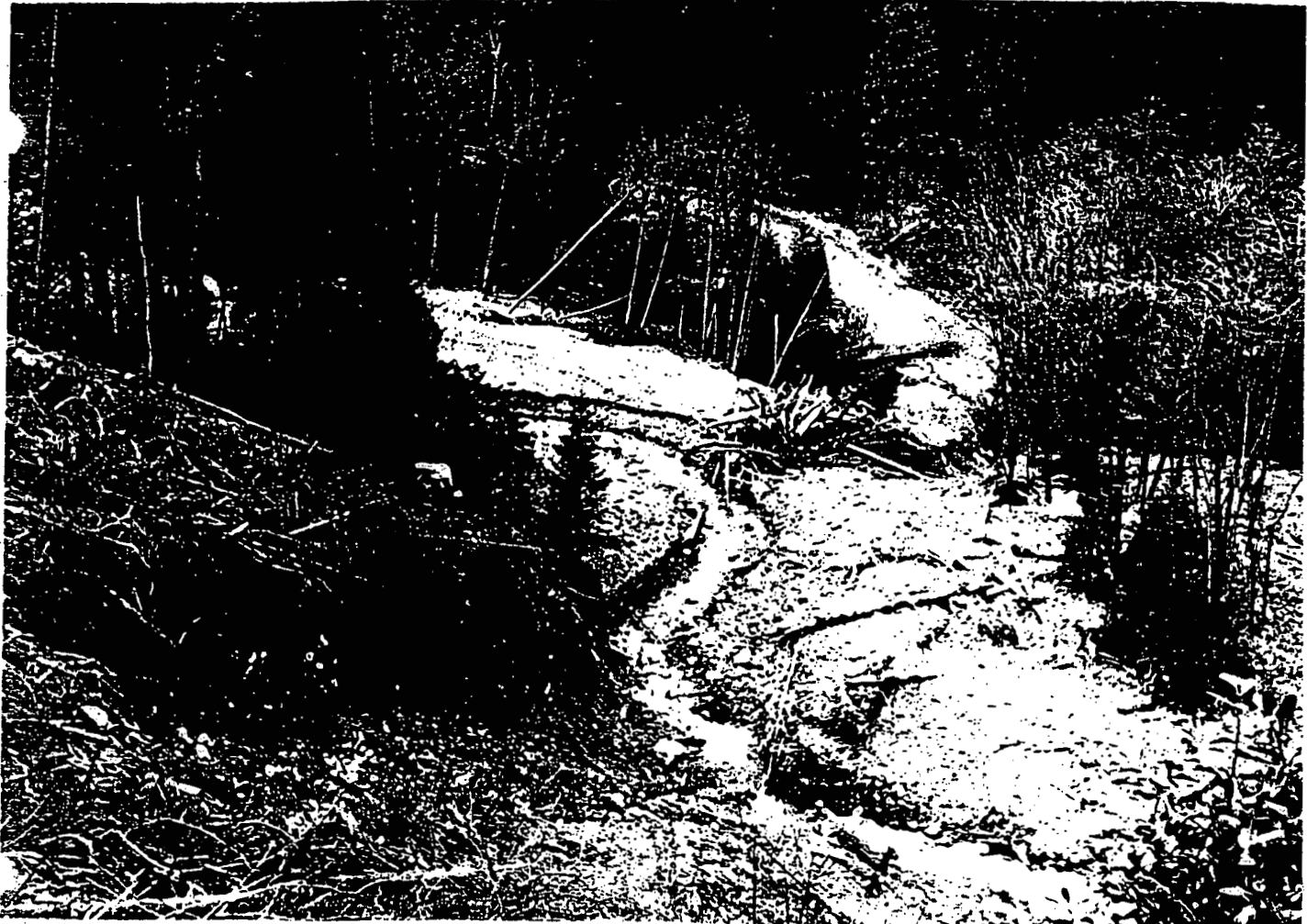
Photo #97-27-6A: Walker Creek road crossing taken out by debris flow. View from the head of a small slump activated by stream undercutting. Road formerly passed along the base of the slump. (J.d.l.F: 4-25-97).
