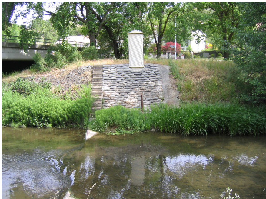
Figure 11--Alamos Creek, near San Jose, California. Gage has a concrete sill, hardened walls, and a traditional stilling well.
