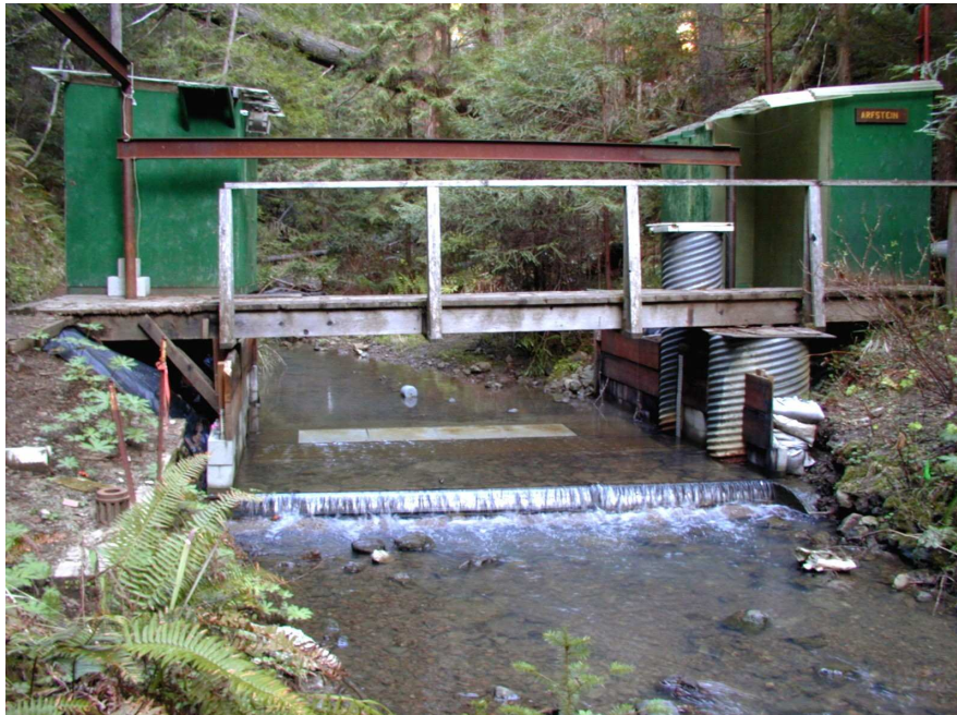
Figure 10-- Rated section with steel sill and side walls in North Fork Caspar Creek, California.
