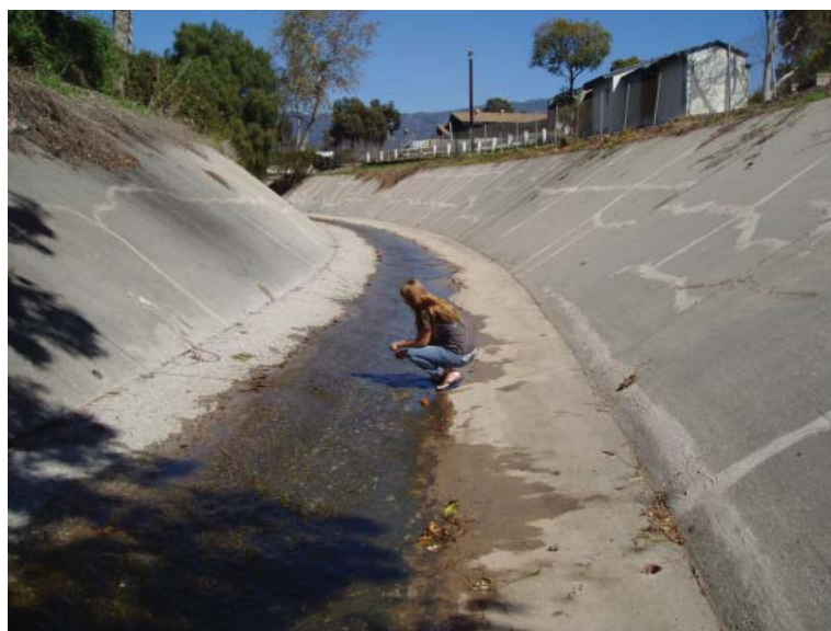
"Hardened" sites such as SJ1 lack many of the characteristics of more natural streams. They typically have little to no riparian cover, and lack rocky or sandy bottoms and banks.
