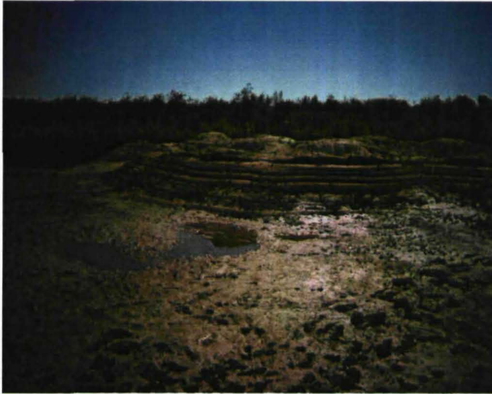
PHOTO 7: Large Lower Lake at the Stockpile Location
