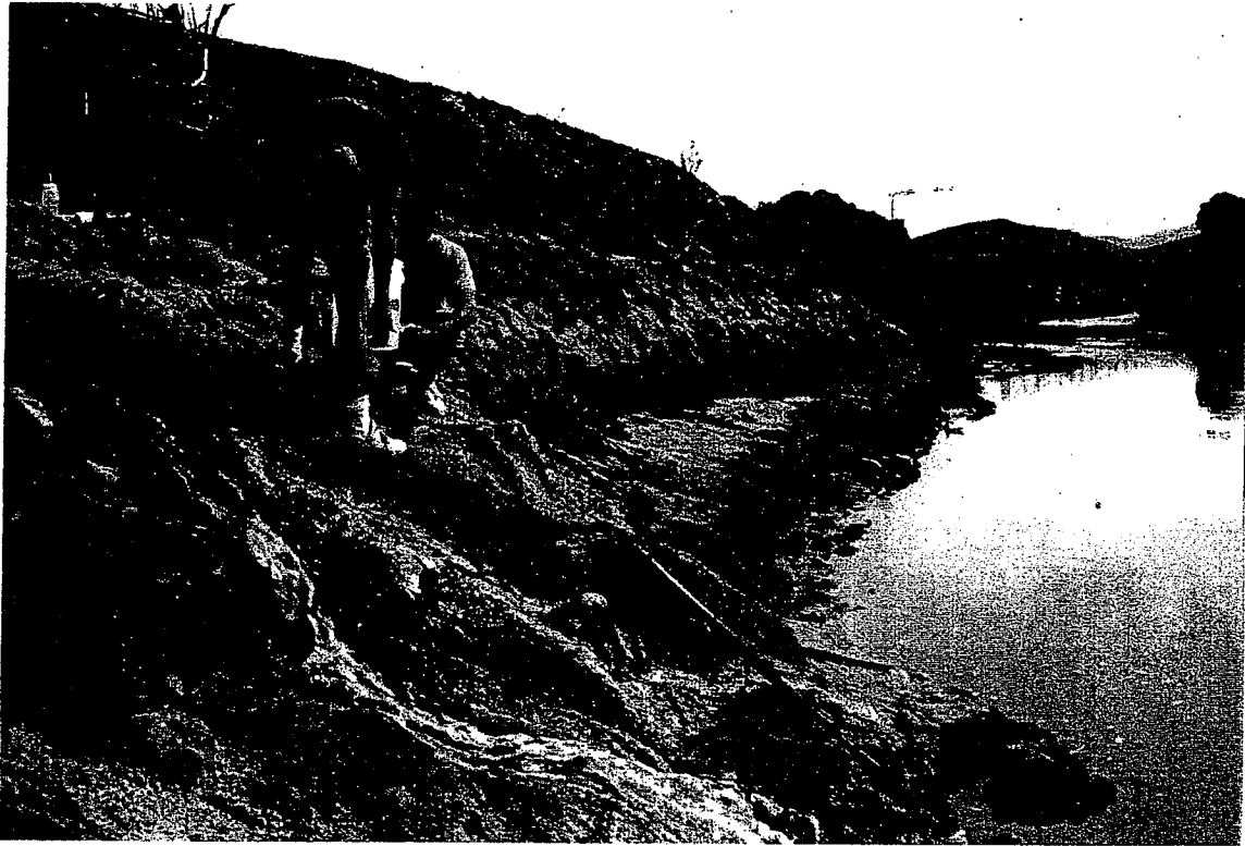
C-3 CONEJO CREEK AT HOWARD ROAD BRIDGE. NOTE AGRICULTURAL DISCHARGE AT LEFT CENTER AND IN FOREGROUND. THE CAMARILLO POTW IS IMMEDIATELY UPSTREAM OF THIS SITE.
