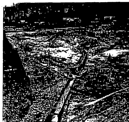
Figure 3. Gravel deposits were washed into sluices (from center to lower part of figure) where gold was recovered.
