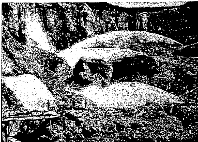
Figure 1. Monitors (water cannons) were used to break down the gold-bearing gravel deposits with tremendous volumes of water under high pressure. Some mines operated several monitors in the same pit. Malakoff Diggings, circa 1860.
