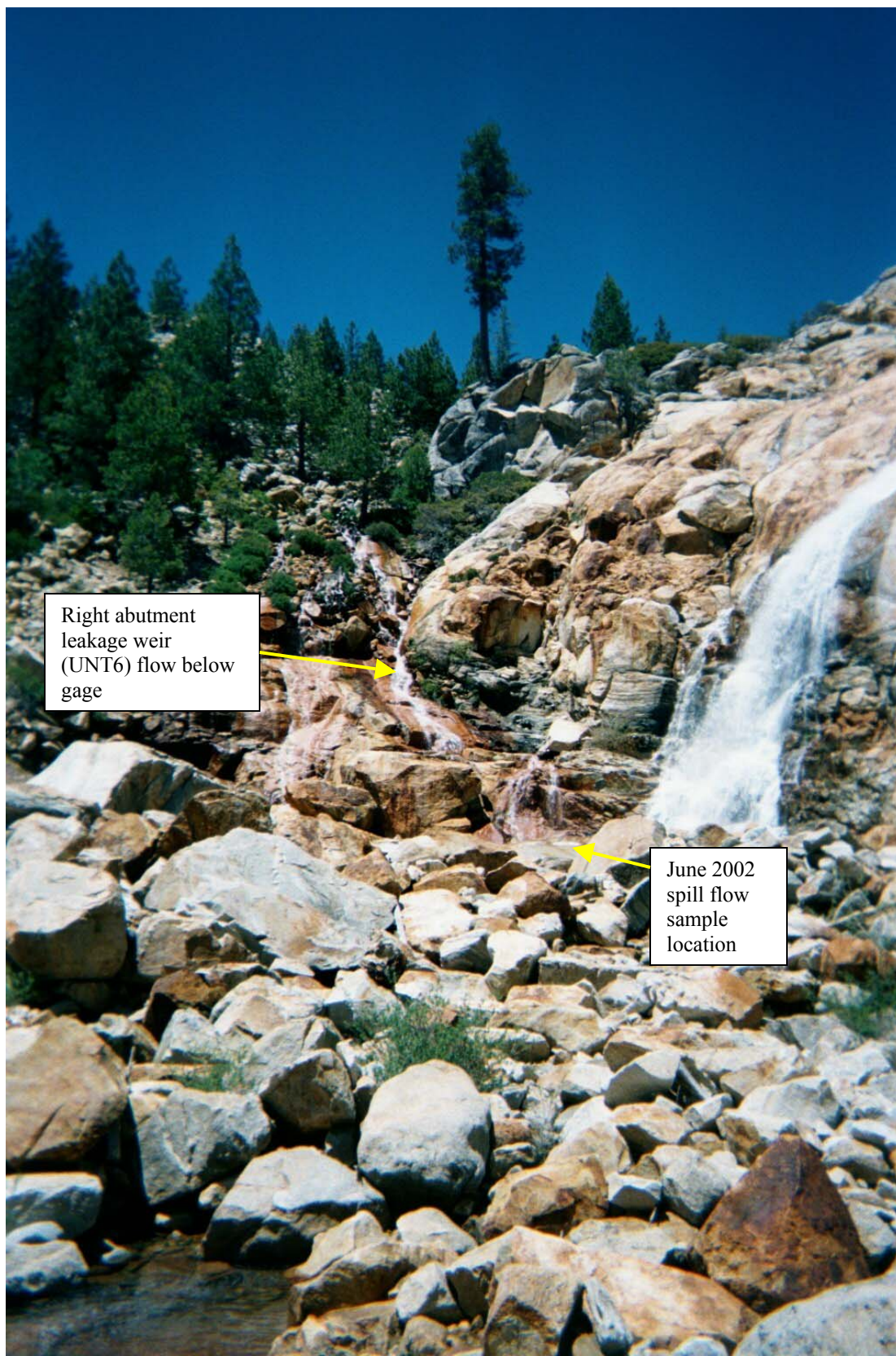
Photo 5. Right abutment leakage weir (UNT6) flow and bottom of spill flow at point of convergence (June 2002)
