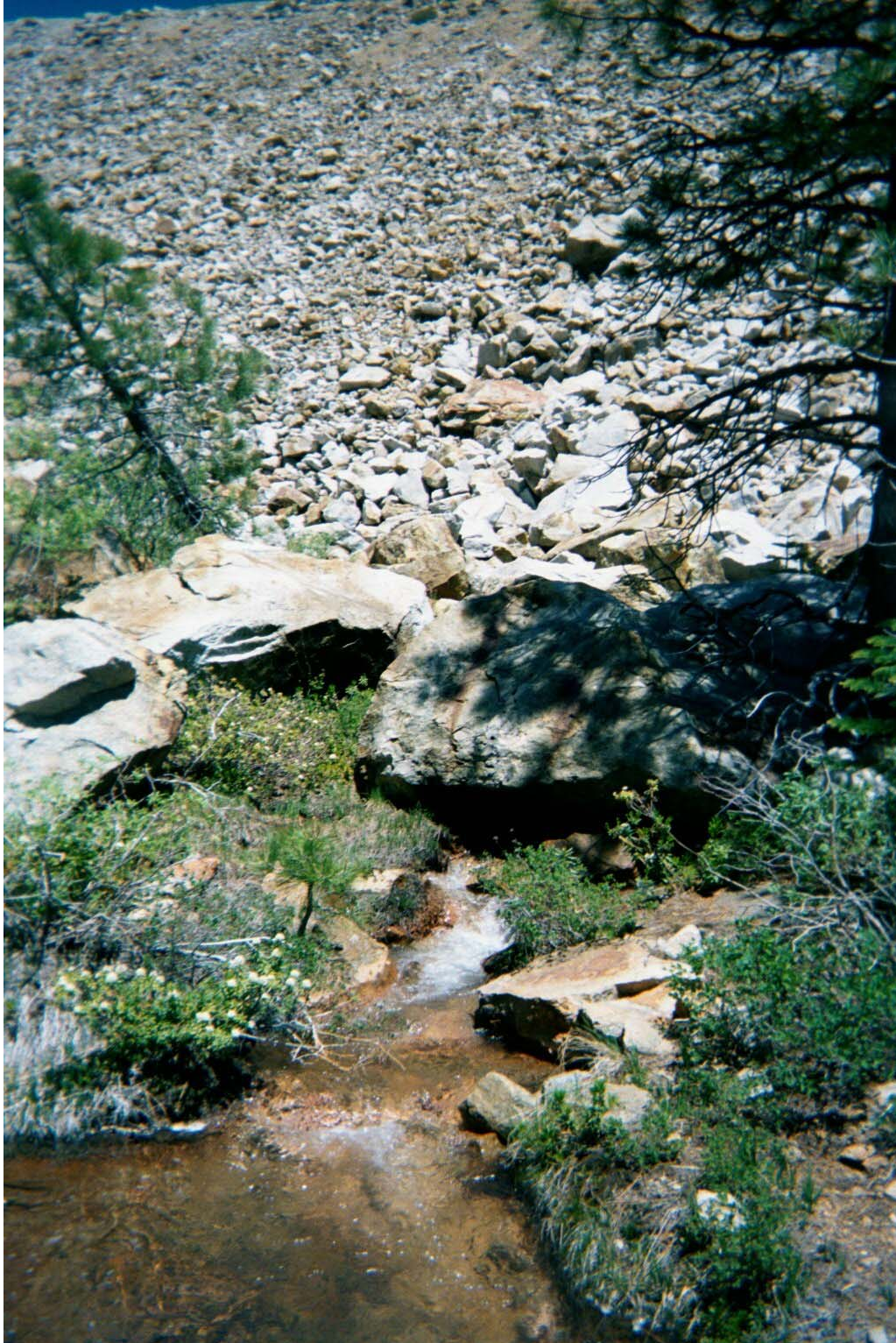
Photo 3. Left abutment leakage weir source (UNT8a) at dam face above the gage (June 2002)
