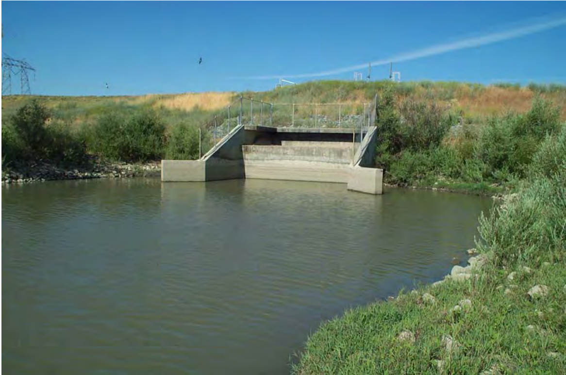
Cache Creek a) low-flow outlet, b) overflow spillway
