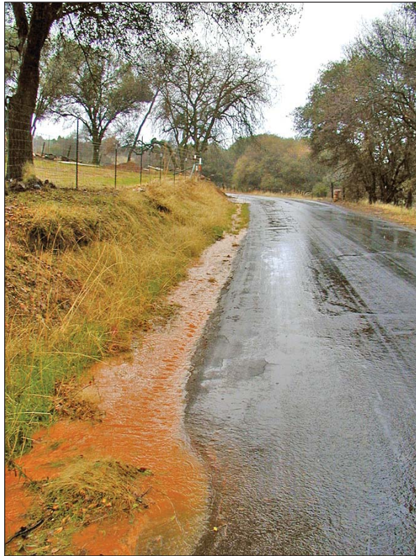
PHOTOGRAPH A. Evidence of sediment-laden runoff being conveyed along a roadside ditch.
