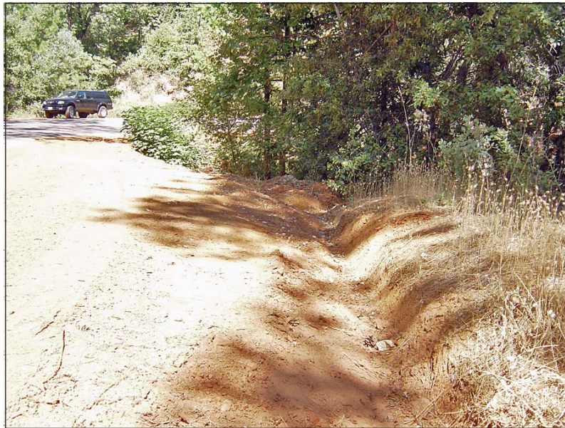
SCR-18. Small tributary to Powerhouse Creek (which drains to Phoenix Lake and then to lower Sullivan Creek). Looking upstream (top), small cascading (could be colluvial) channel typical of the steep headwater streams draining the northern half of the Upper Sullivan (or Phoenix Lake in this case) watershed. Roadside ditch (bottom) delivering weathered material (likely mostly clays, silts, and fine sands) to the hillslope and channel.
