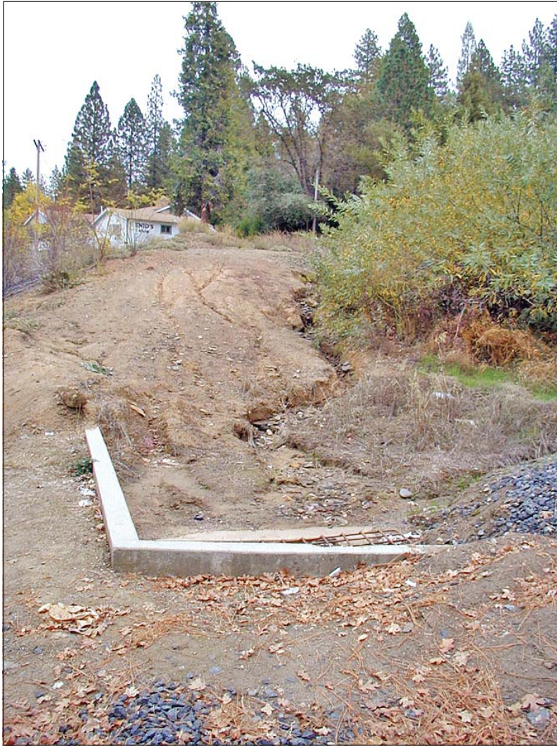
PHOTOGRAPH C. Gully formation below State Route 120 in Groveland.
