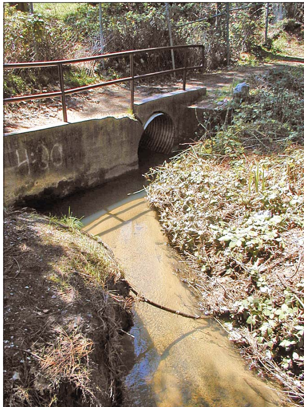
TWH-1. Small reach of Twain Harte Creek parallel to Epscol Park. Upstream end (top) is fed by two large culverts; downstream end (bottom) is backed-up by another culvert under the footpath. Morphology is highly altered, significant accumulation of sand within this reach and evidence of recent bank erosion and channel incision.
