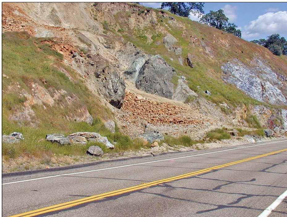
PHOTOGRAPH F. Active rock fall above Jacksonville Road; east of Don Pedro Reservoir.
