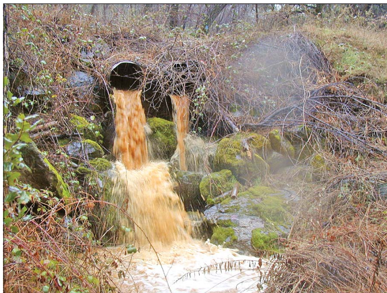
PHOTOGRAPH B. Highly turbid discharge below a storm drain outfall.
