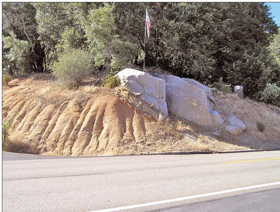
Boulder remnant within granitic weathering zone along Phoenix Lake Road near Oakhaven Lane. Rills deliver eroded sediment to roadway and Sullivan Creek.
