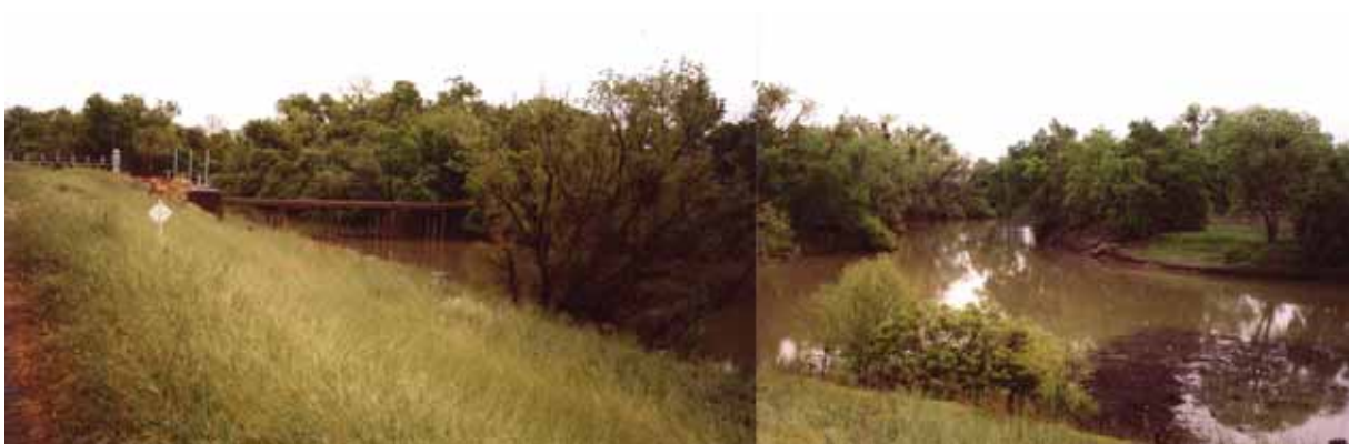
PHOTO 4 SSB: Sacramento Slough Bridge
