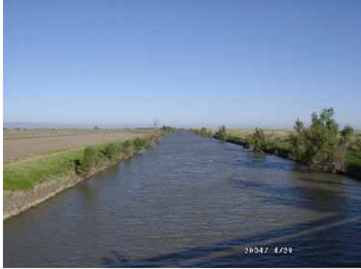
PHOTO 1 CBD1: Colusa Basin Drain #1
