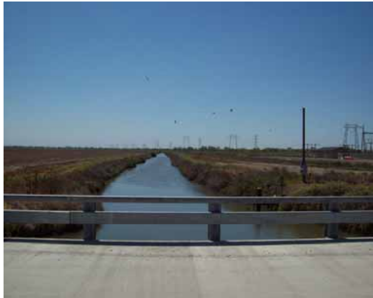
PHOTO 7 H: Obanion Outfall
