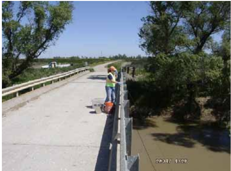
PHOTO 2 CBD5: Colusa Basin Drain #5
