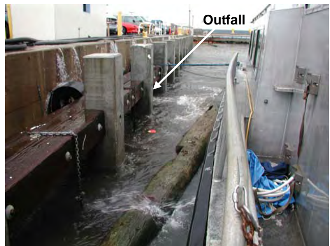
Fig. 3. RV ECOS tied up along quay wall outside OF14. The sensors and pump intake were directly in line with the outfall. Note sheet runoff over quay wall.
