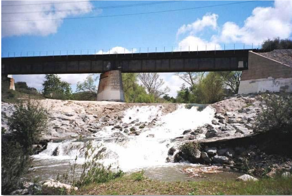
Figure 2. Metrolink rail crossing concrete and aggregate structure (looking upstream) on Trabuco Cr. several miles downstream of CNF land in San Juan Capistrano, CA. This approximately 30-foot tall structure is a barrier to all life stages of southern steelhead trout. The barrier height is increasing due to continual vertical scour at the base of this large artificially hardened streambed structure. Photo from CDM, et al. 2007.
