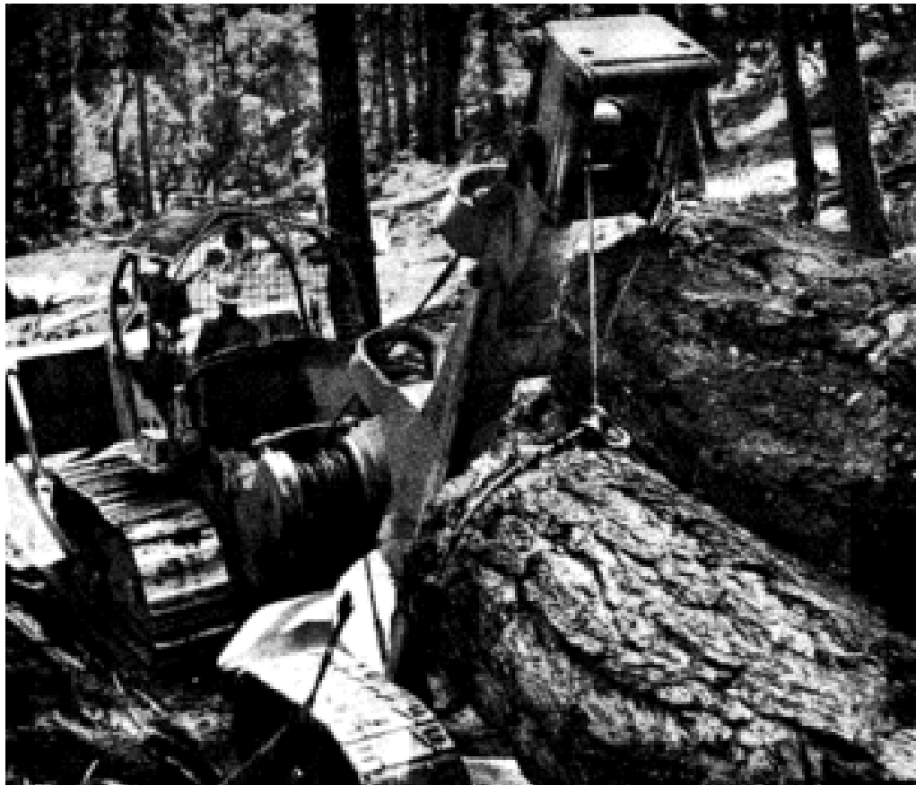
Figure 31. Tractor arch operations.
