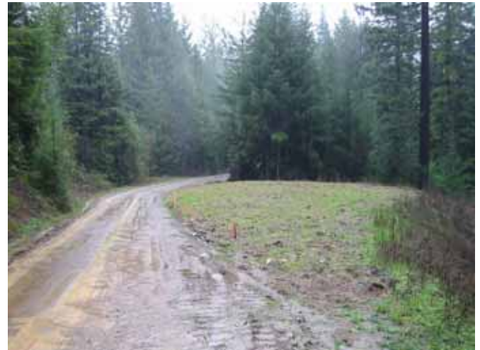
Figure 38. Reclaimed landing on mainline road.
