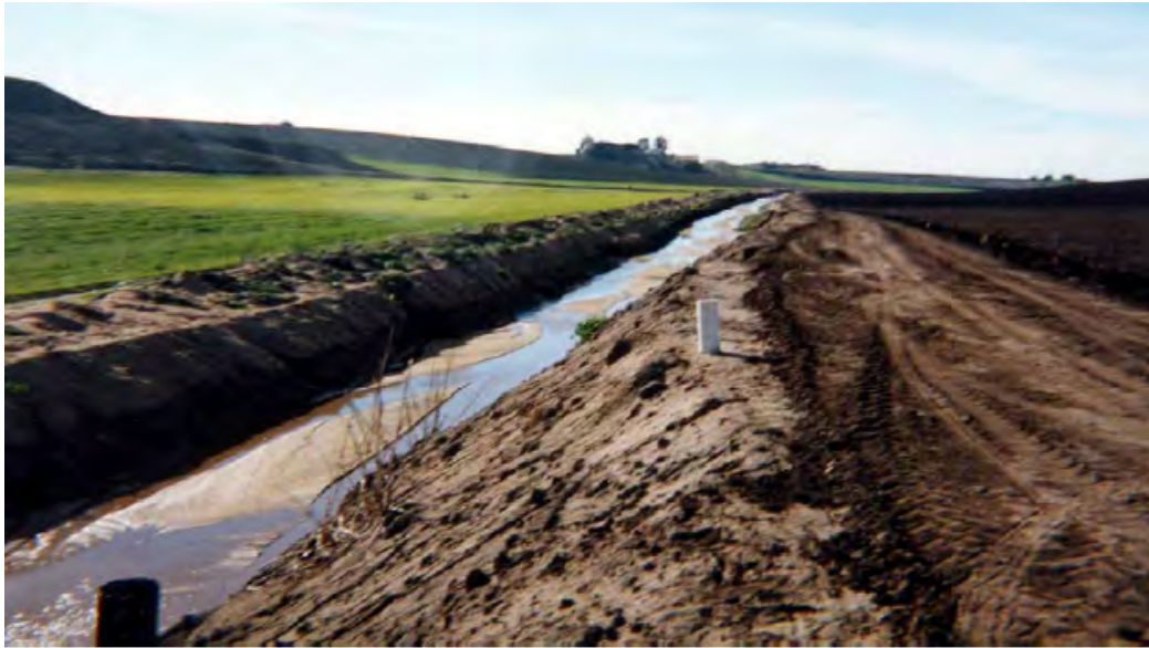
Figure 5. Lower Santa Rita Creek photo taken from Casagrande and Watson (2006, Fig 4-17) shows this stream is completely channelized and excavation activities appear to have increased erosion risk.
