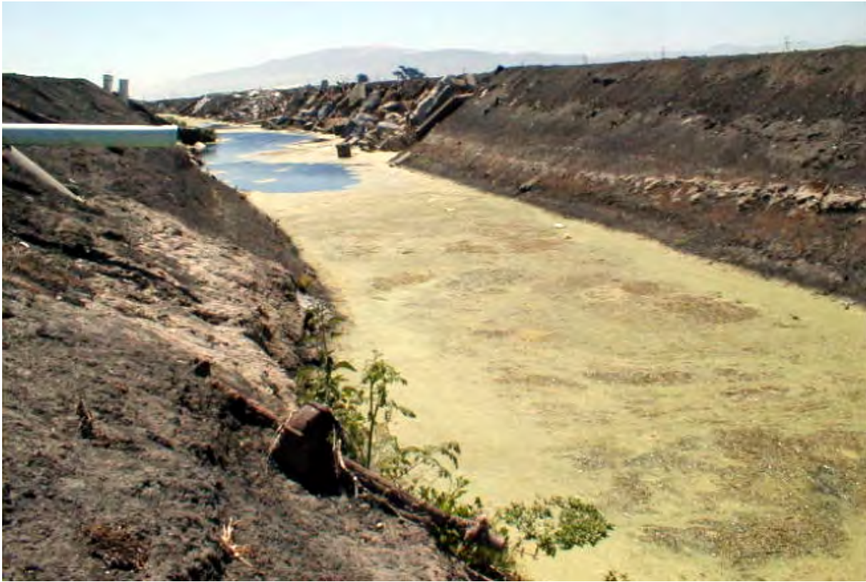
Figure 9. Photo of Reclamation Ditch at San Jon Road with nuisance algae bloom induced by low flow, nutrient loading and lack of shade. Photo from Casagrande and Watson (2006).
