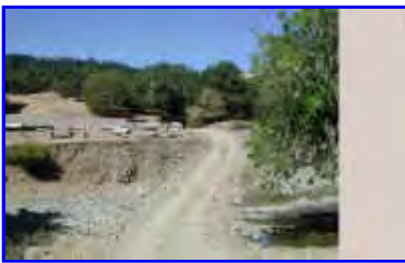
Figure 5. This is a view of temporary road blocking Beebe Creek near Highway 128 above its convergence with Rancheria Creek. This crossing formed a dam which caused flows to pond on the upstream side and to block downstream flows. Dry reaches constitute a constraint on salmonid production whether the origin of flow loss is diversion, aggradation or changes in runoff patterns as a result of cumulative watershed effects. Photo by Pat Higgins, 9/21/01.
