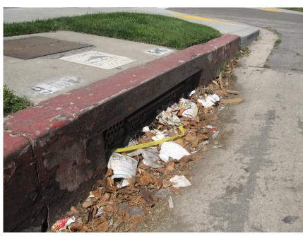
Figure 9 **Gross Solids Protruding Through GRSD Screen**
