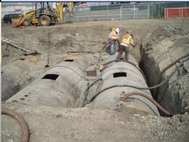
Photo 1: Excavation of three 10,000-gallon USTs
