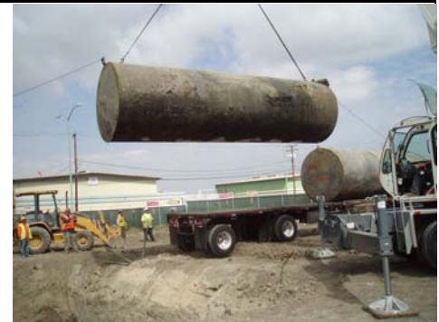
Photo 2: Removal of three 10,000-gallon USTs
