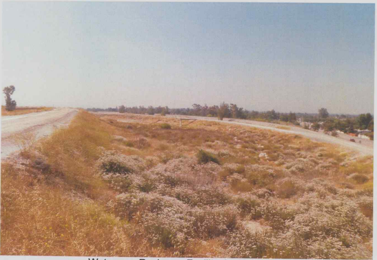
Waterman Recharge Facility, looking East.
