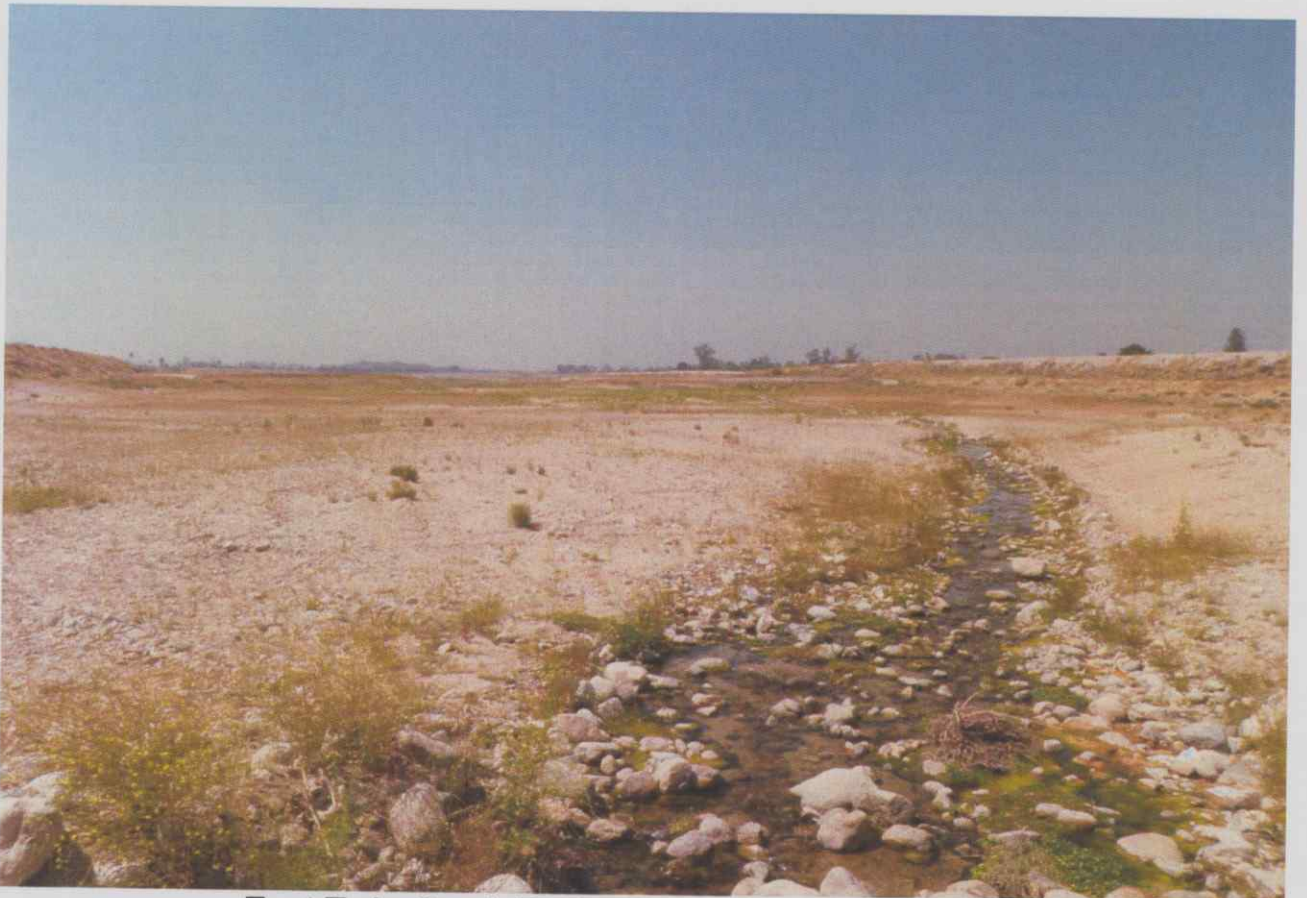
East Twin Creek Recharge Facility, looking South.
