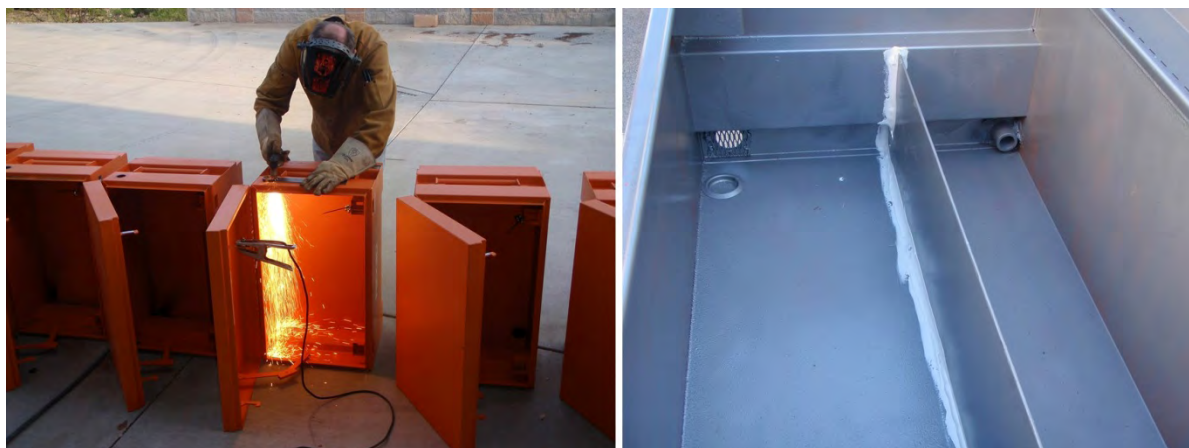
Figure 5. Modifications to the acoustic receiver boxes for the 2009 VAMP study. Left picture: plasma cutting ventilation holes. Right picture: inside of the modified job box showing the water bath compartment and drainage pipe on the right and the dry compartment on the left for housing the data logger and ventilation hole.
