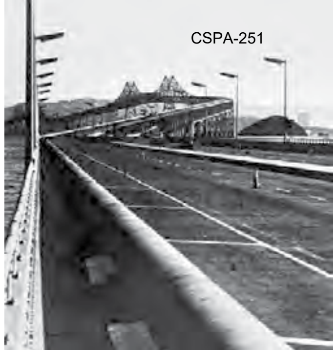
Emergency pipeline constructed during 1976–77 drought to bring water to southern Marin County.
