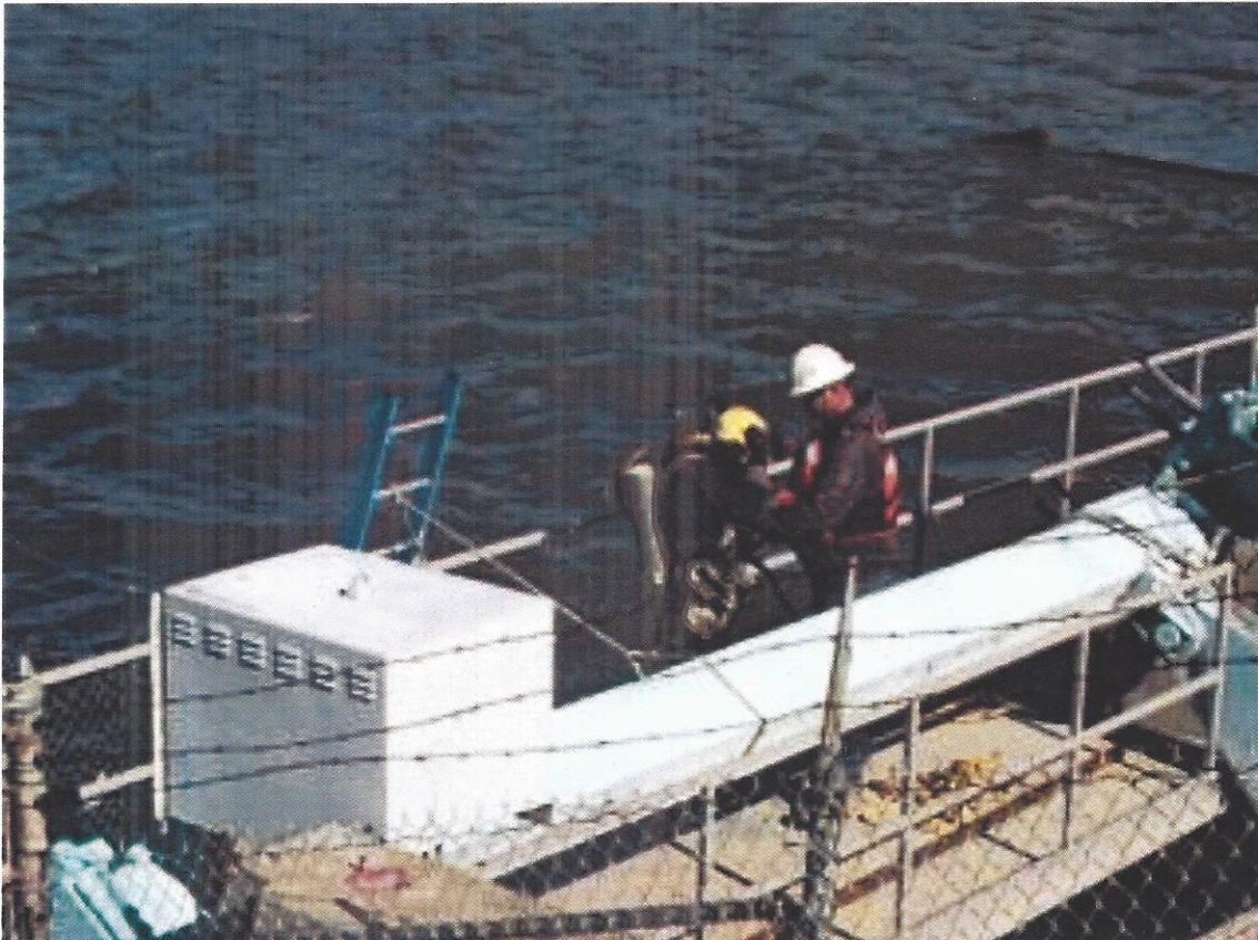
Photo 2: View of the diver getting ready to enter the water from the scaffolding at bay 1.
