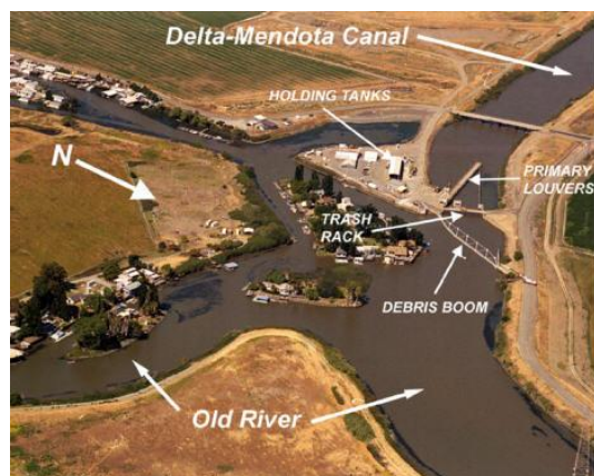
The CVP's Tracy Fish Collection Facility
