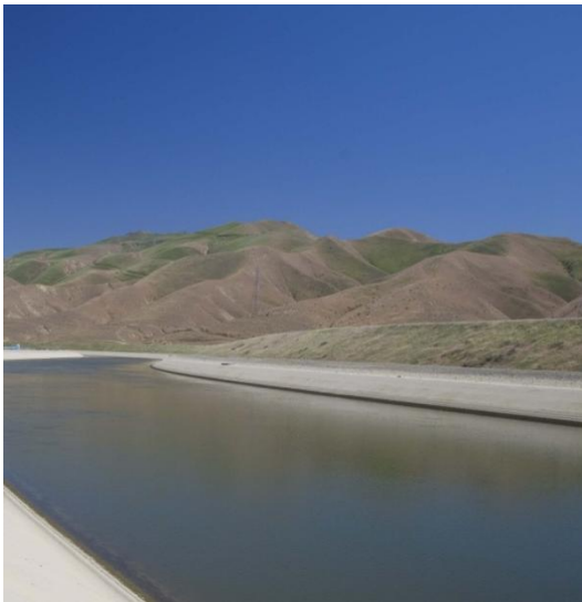
Aqueduct of the State Water Project
