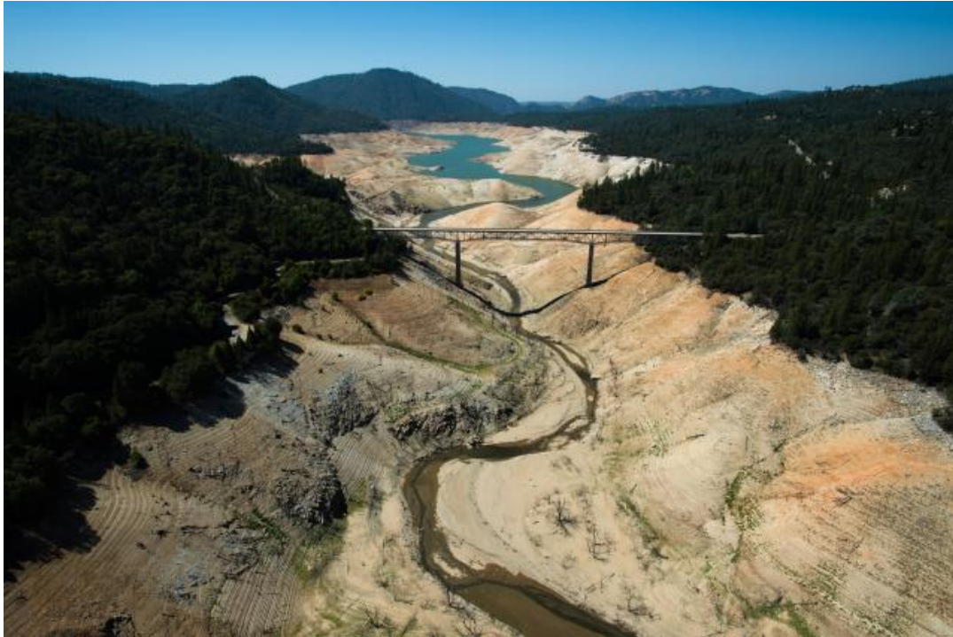
South Fork of Lake Oroville, California's second largest reservoir, on Sept. 5, 2014
