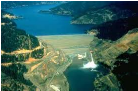
Trinity Dam shortly after completion in 1963.
