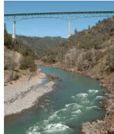
Ben Furtado/Auburn Journal file photo The Foresthill Bridge was built as part of the Auburn dam construction project in the early 1970s as a bridge over what would have been a reservoir inundating much of the American River canyon in the Auburn area. The point where the concrete pillars meet the bridge’s steel trusses would be the high-water mark.
