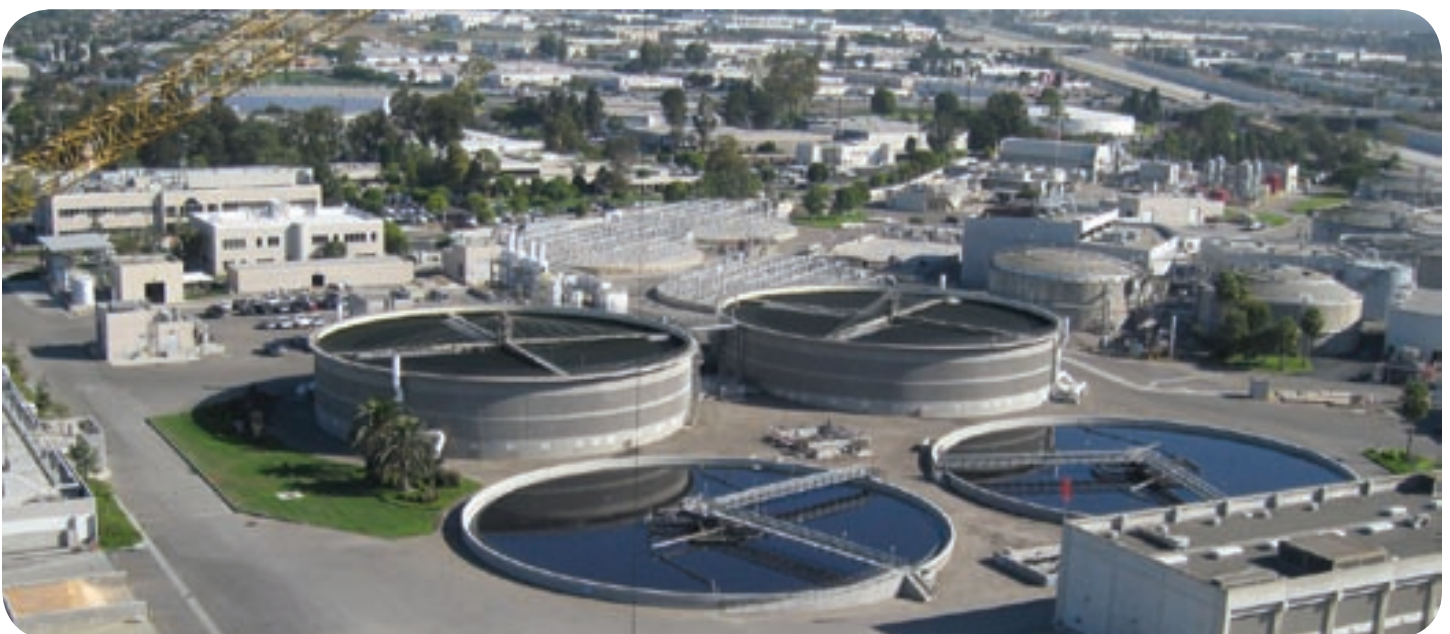
The Orange County Water Recycling facility.
