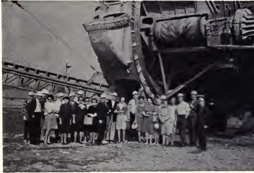
Fifth Annual Inspection of the work at Oroville Dam. Director of the Department of Water Resources, principle staff and their wives, standing near "the monster." March 27, 1966.
