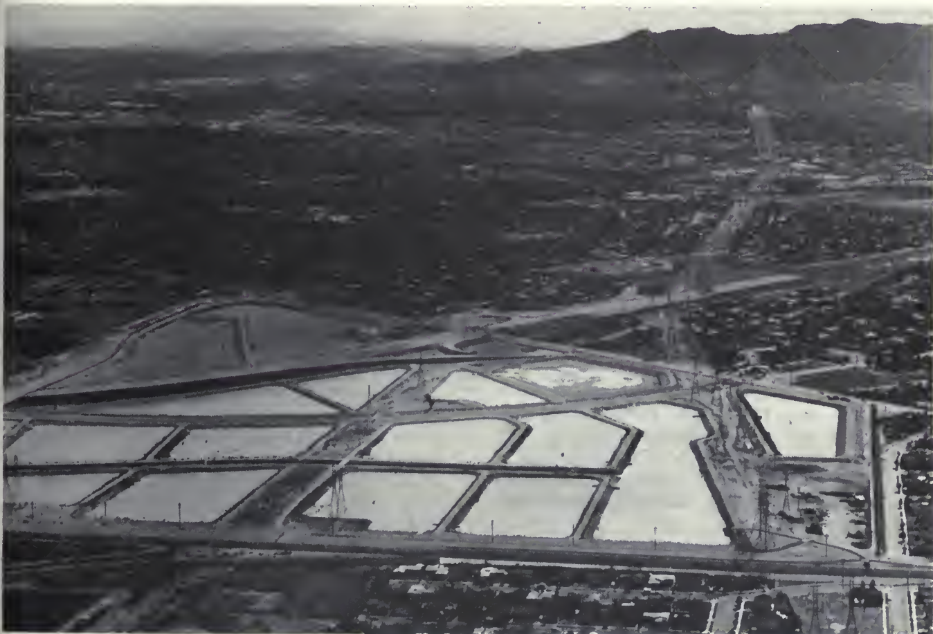
Tujunga spreading grounds in San Fernando Basin.
