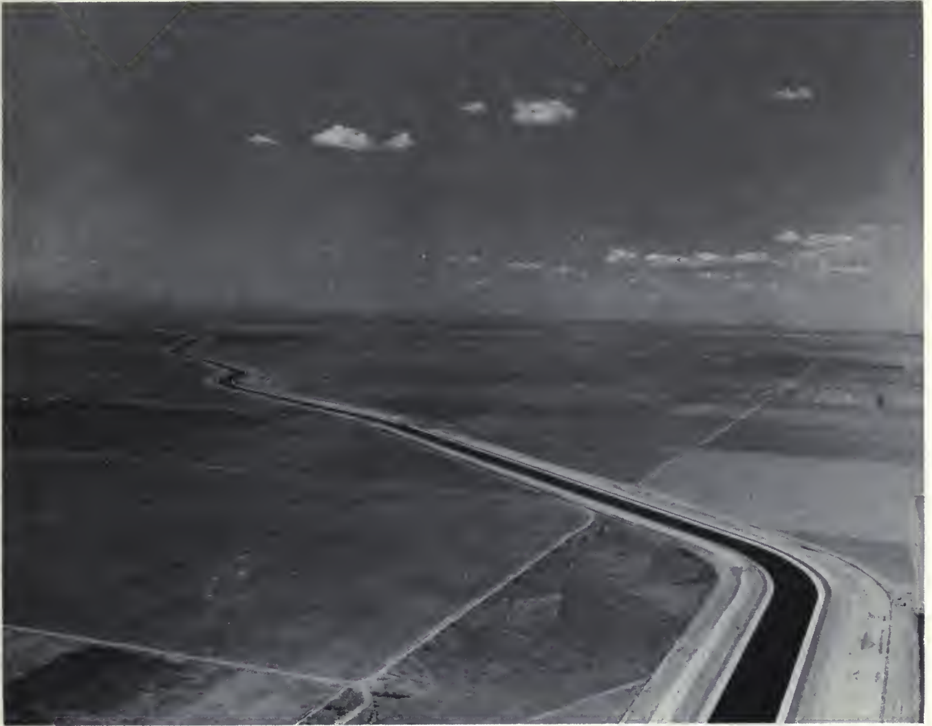
The California Aqueduct transports water from the Delta to State Water Project service areas.
