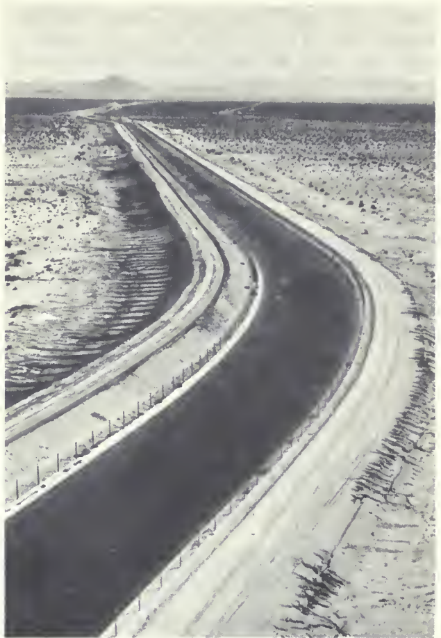
Open canal portion of the Colorado River Aqueduct.
