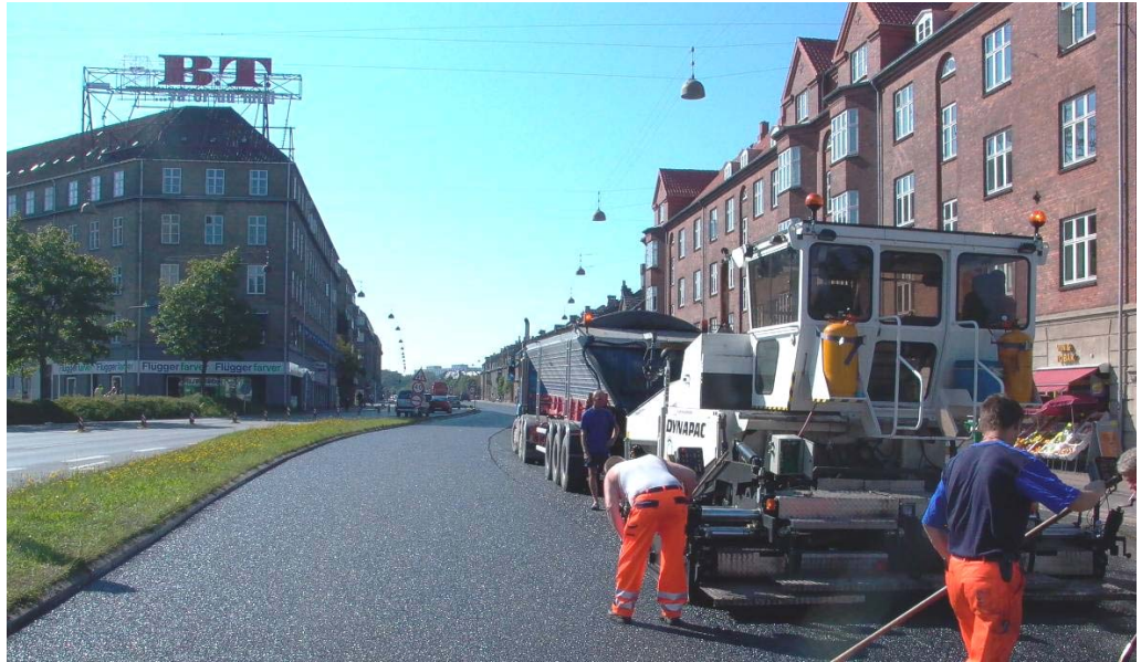
Figure 6.6. When the pavement on an existing highway has to be replaced, the road administration might consider using a new noise reducing pavement type. Here noise reducing two-layer porous asphalt is applied on a highway in a densely built up area in the municipality of Copenhagen.
