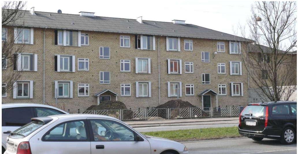
Figure 6.9. Noise reducing window constructed as a "noise shutter" that makes it possible to open the window. Placed in front of bedrooms and living rooms facing the highway (photo Allan Jensen, Rambøll).
