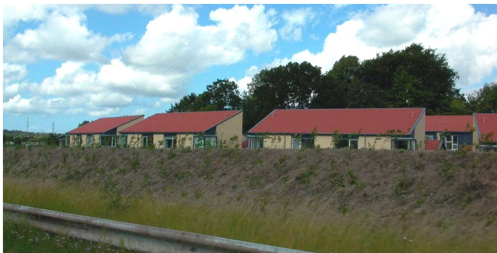
Figure 7.1. Earth embankment constructed at the same time as a new housing district to reduce the noise from an existing road at the houses and the gardens at Kvistgård, Denmark.
