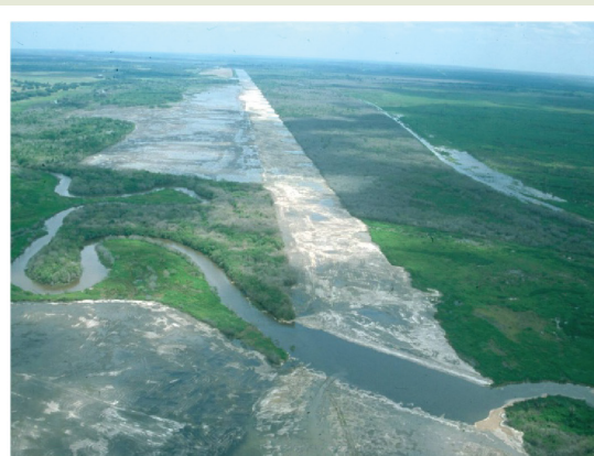
February 9, 2001, photo of implemented phase one Kissimmee River Restoration Project showing the backfilled canal, degraded soil area, remnant river channel, the connector channel, and wetland areas.
