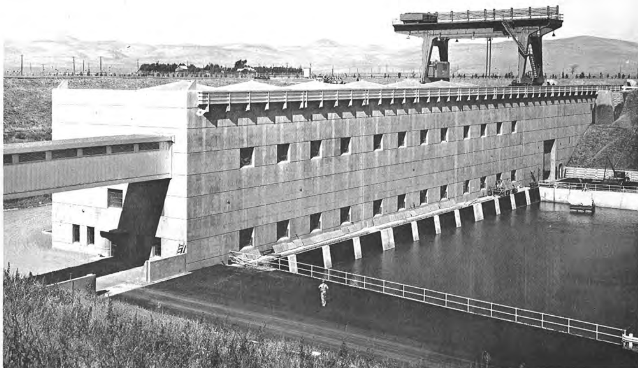
TWO EXISTING FEATURES OF THE CENTRAL VALLEY PROJECT, TRACY PUMPING PLANT (ABOVE) AND DELTA-MENDOTA CANAL (BELOW), WOULD LIFT WATER FROM THE SACRAMENTO - SAN JOAQUIN DELTA AND CONVEY IT 67 MILES SOUTHWARD TO THE SAN LUIS AREA
