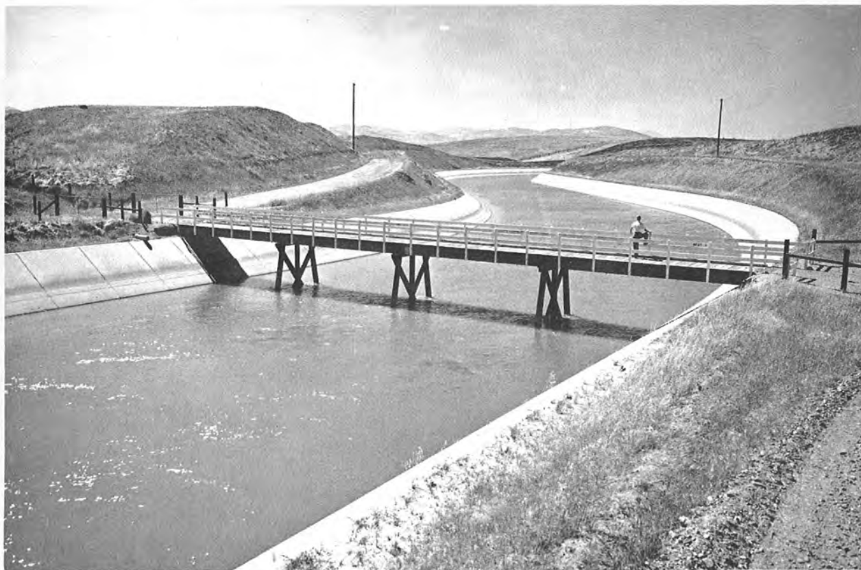
TWO EXISTING FEATURES OF THE CENTRAL VALLEY PROJECT, TRACY PUMPING PLANT (ABOVE) AND DELTA-MENDOTA CANAL (BELOW), WOULD LIFT WATER FROM THE SACRAMENTO - SAN JOAQUIN DELTA AND CONVEY IT 67 MILES SOUTHWARD TO THE SAN LUIS AREA
