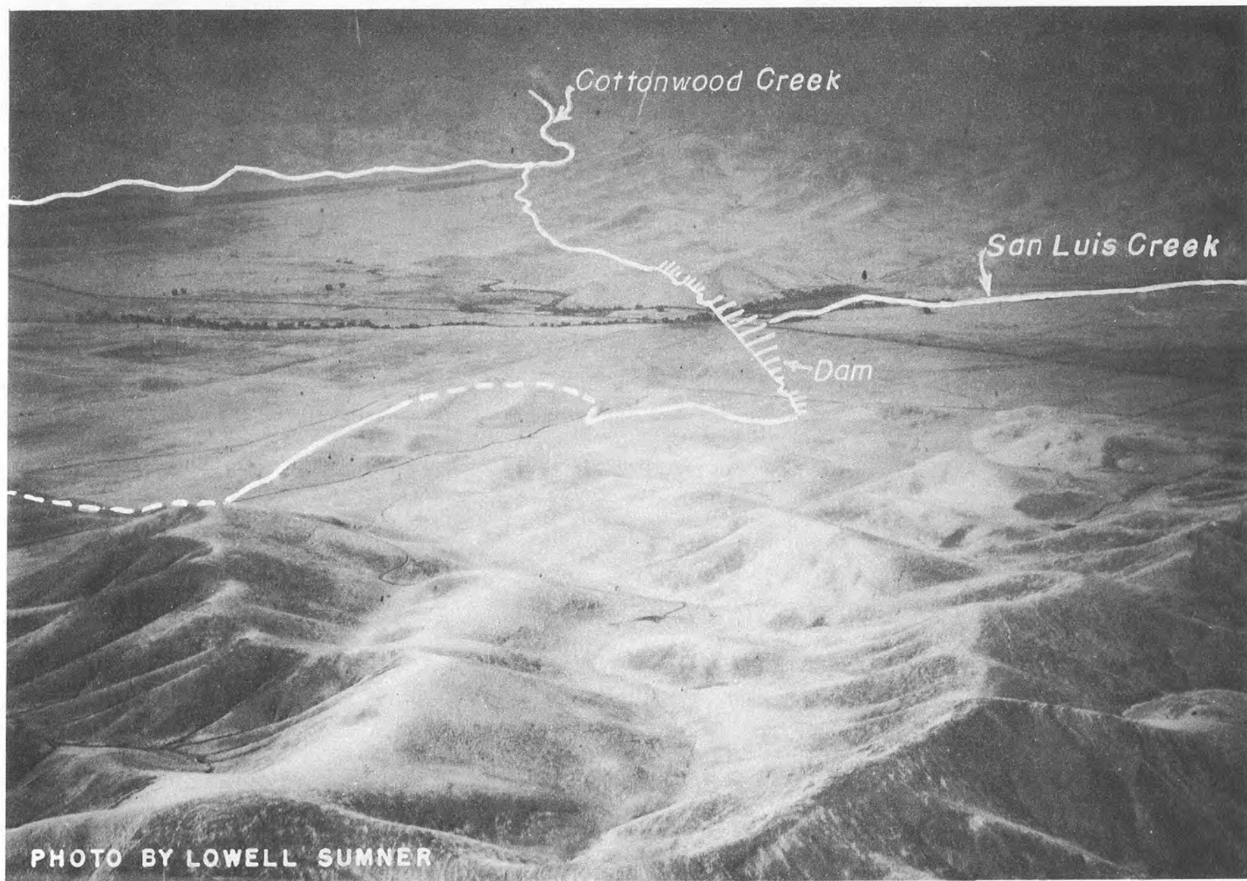
AERIAL VIEW NORTHWEST OVER SAN LUIS DAM SITE
