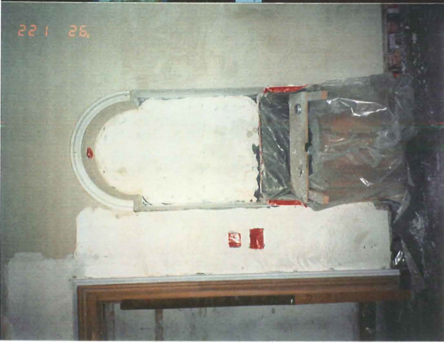
During Restoration - See new plaster "married" into original
