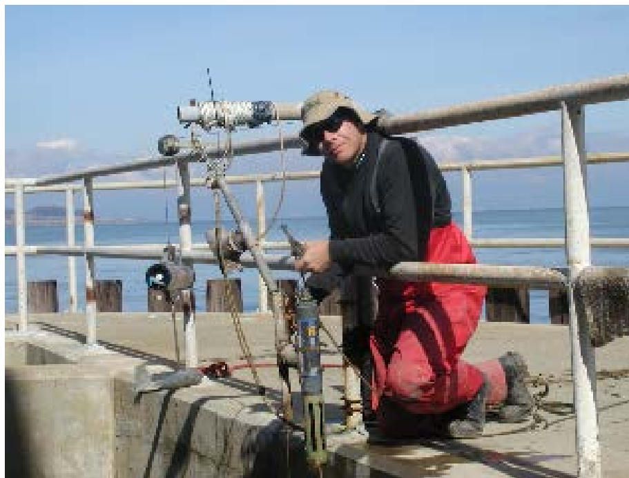
Figure 3-5 Example of USGS WQ Monitoring Station (using YSI 6920V2 internal logging Sonde)
