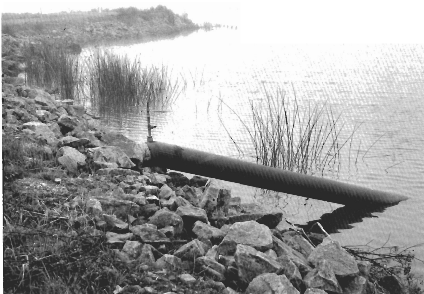
Figure 14.—Irrigation water for cropland in the Delta area is commonly siphoned from the adjacent sloughs and piped through levees to the fields.
