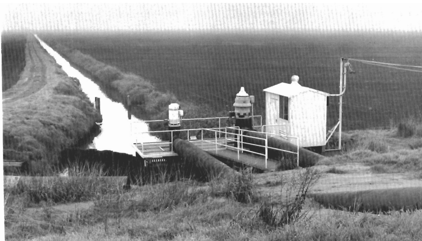
Figure 11.—A pump in the Delta area, where excess water is pumped from the main drainage ditches and returned to a river or slough across the levee.
