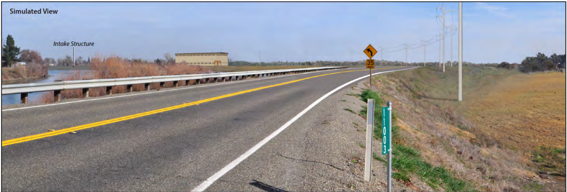
Figure 17-78 Existing and Simulated Views of Intake 4 East from SR 160 (Alternatives 1A, 1B, 2A, 2B, 6A, and 6B)
