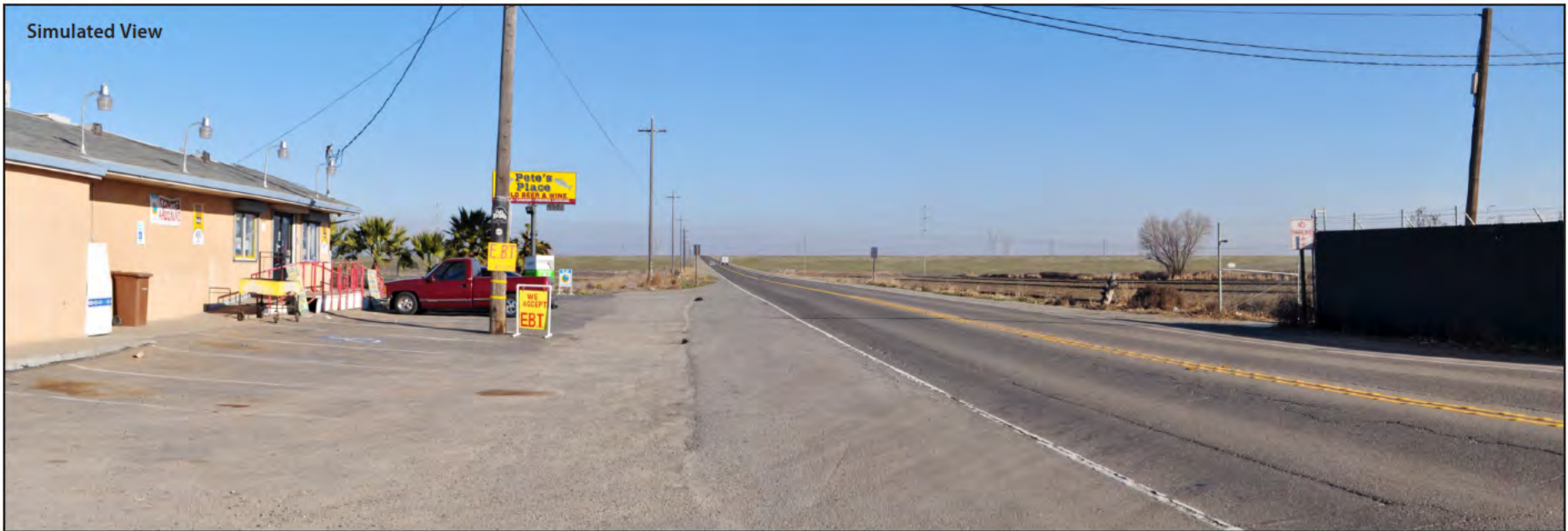
Figure 17-83 Existing and Simulated Views of the East Canal from SR 4 (Alternatives 1B, 2B, and 6B)
