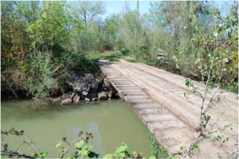
Railcar crossing without concrete abutments at the Island, YBWA. This crossing is recommended for replacement with concrete abutment railcar crossing. (See Figures A-10a and A-10b).
