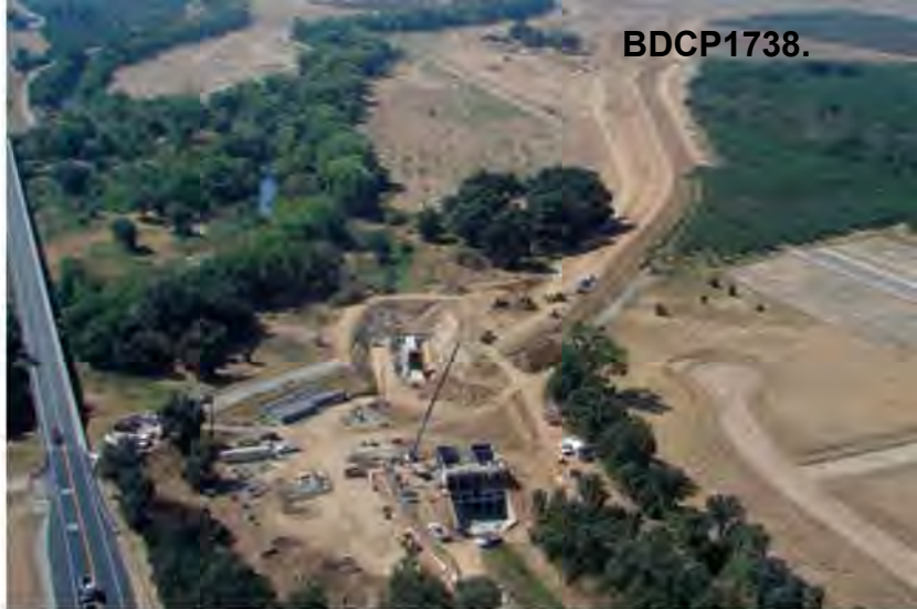
Setback levee being constructed near Bear River
