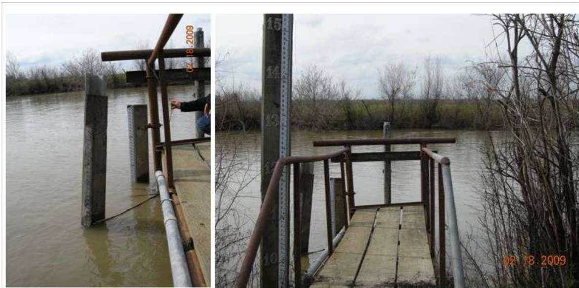
Figure 5.A.A.4-7. Photos taken February 18 2009 between 1:45 - 2:00 pm downstream of the Lisbon Weir. Stage approx. 7.4 ft NAVD88. Flows were 1982 cfs at 13:45 and 1943 at 14:00 (DWR unpublished data)
