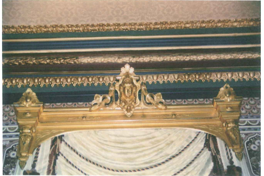
Crown Molding Restored 1992
