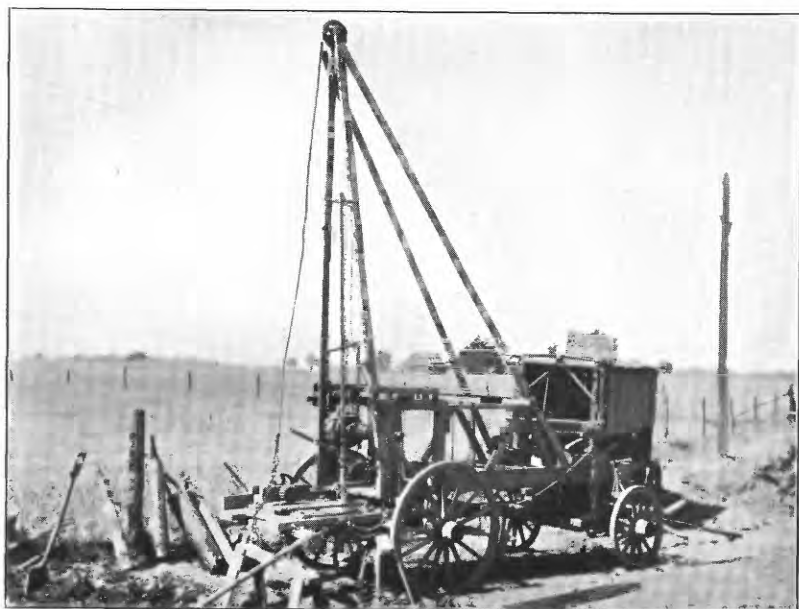
A. SMALL BORING RIG OR WELL AUGER.
