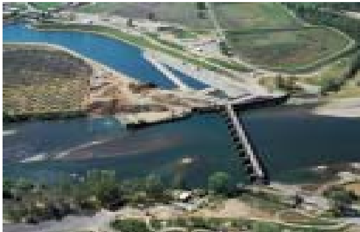
The Red Bluff Demonstration Pump Project fixed fish passage problems at Red Bluff Diversion Dam.
