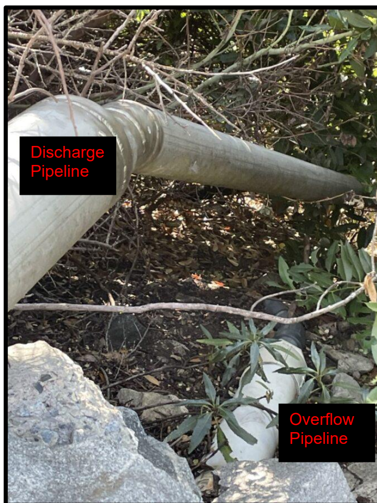
12. Spring 2: Looking at discharge pipeline and plastic overflow pipe
