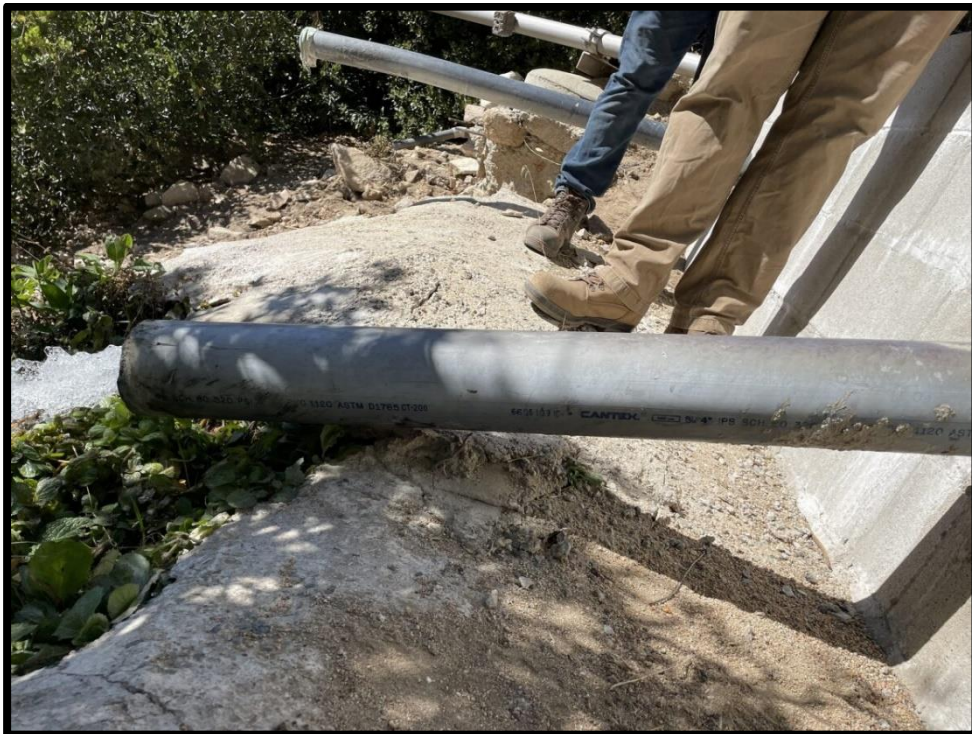
31. Spring 7ABC: Looking at vault overflow pipeline (note flow coming out of pipe)
