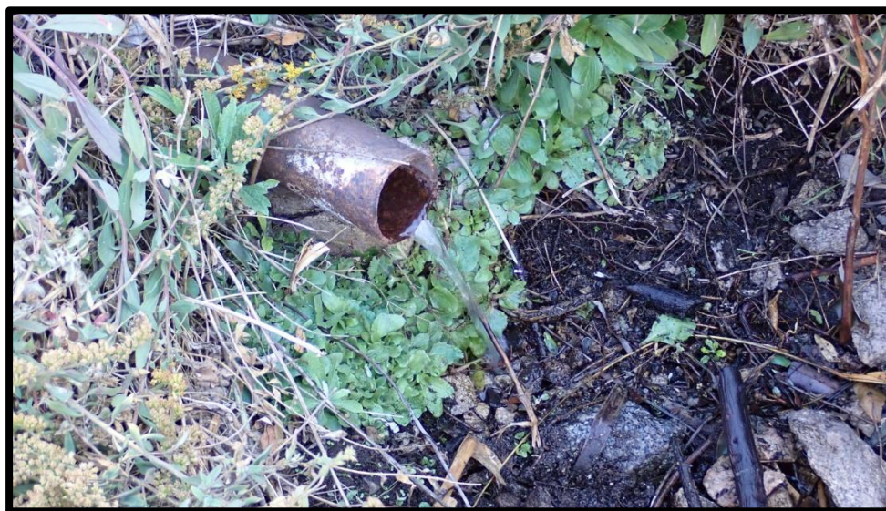
13. Spring 2: Looking at flow out of vault overflow pipe
