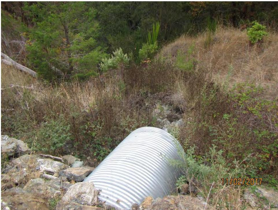
**Figure 14.** Substantial obstruction of the natural flow and alteration of the bed, bank, and channel of an unnamed tributary to Bear Creek and the South Fork Eel River by the placement of a culvert and fill within the channel.
