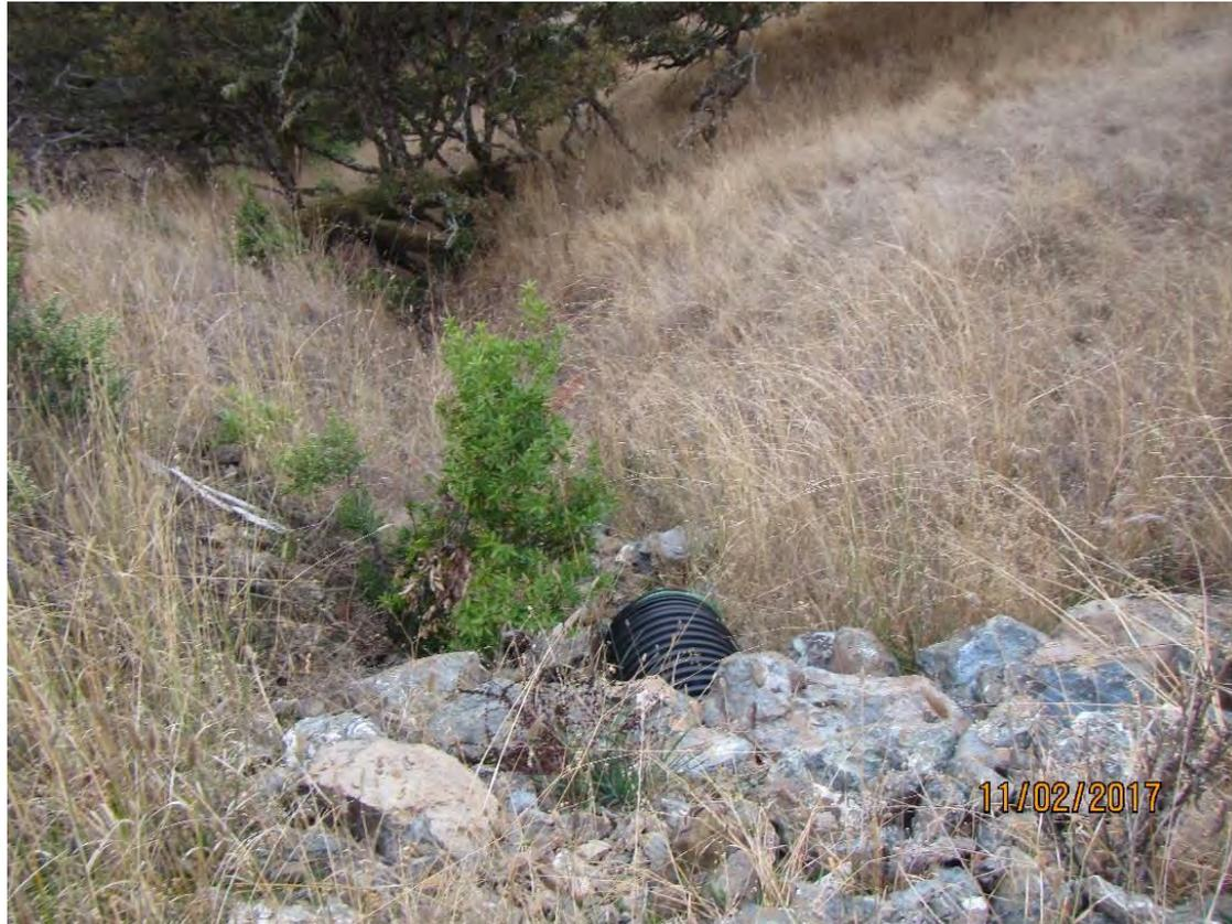
**Figure 15.** Substantial obstruction of the natural flow and alteration of the bed, bank, and channel of an unnamed tributary to Bear Creek and the South Fork Eel River by the placement of a culvert and fill within the channel.
