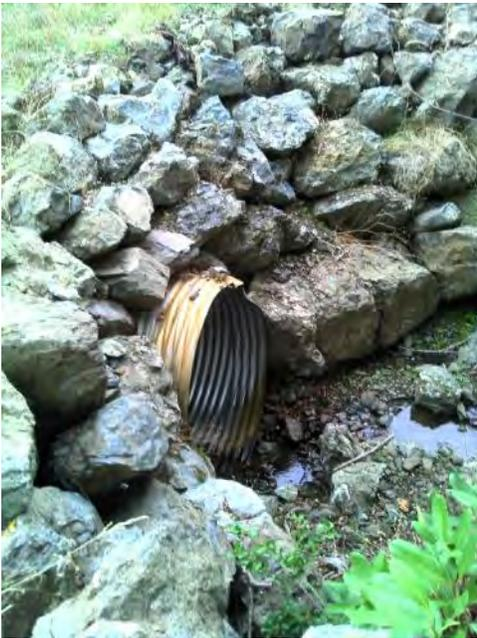
Photo 49: Image of upstream side of stream crossing C6 armoring of streambank of Class II watercourse.
