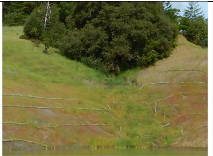
Photo 4: Close up of upgradient topographic swale in Photo 4 showing rills and disturbance of straw wattles.
