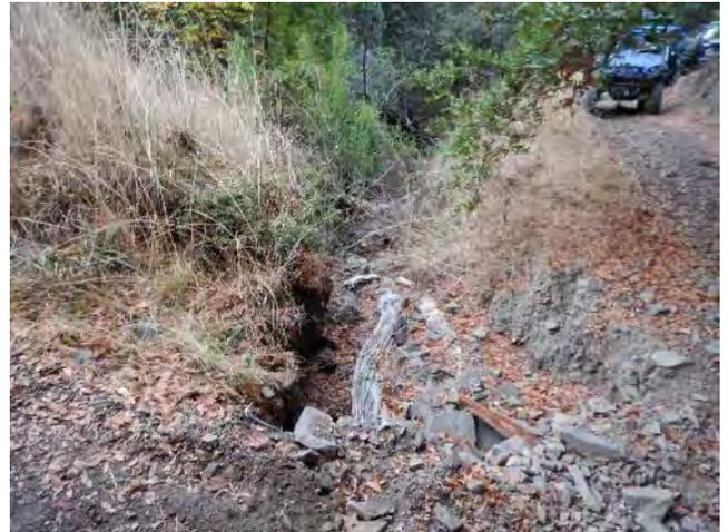
Photo 34: Image of downstream side of stream crossing C1 blocking Class III watercourse and showing erosion of the streambank.
