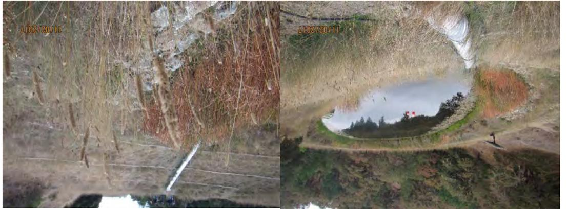
**Figure 4.** Substantial alteration of the bed, bank, and channel to an unnamed tributary to Bear Creek and the South Fork Eel River by placement of rip rap where the Class III channel meets the on-stream pond.
