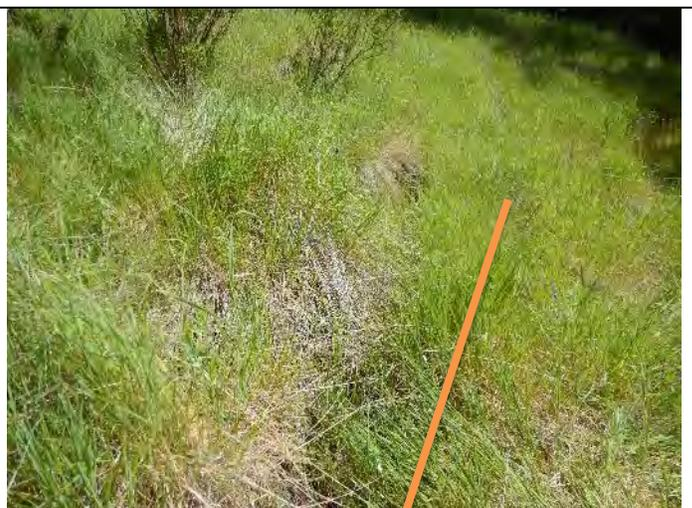
Photo 15: Image of lateral surface cracking below POND2. Orange line is below the lateral crack.
