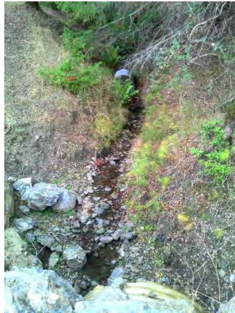
Photo 50: Image of downstream side of stream crossing C6 showing culvert was not placed in alignment with the Class II stream channel.
