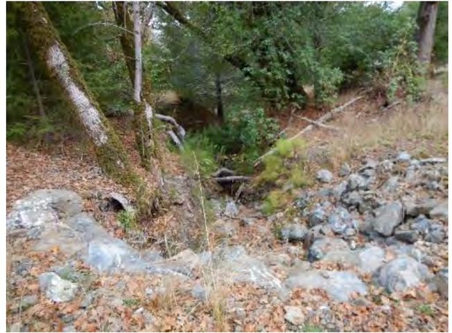
Photo 44: Image of downstream side of stream crossing C3 showing armoring of streambed and streambank.
