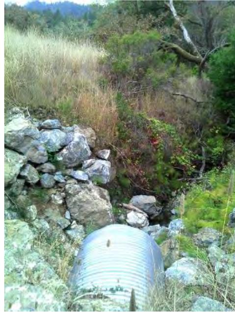
Photo 52: Image of downstream side of stream crossing C7 showing culvert was not set to the grade of the stream channel.
