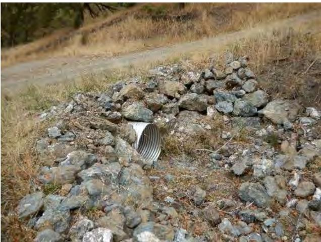
Photo 45: Image of upstream side of stream crossing C4 showing armoring of streambed and banks.
