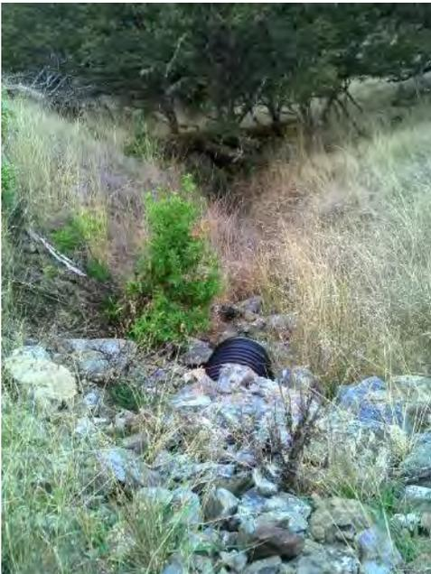
Photo 53: Image of downstream side of stream crossing C8 showing armoring of stream channel.
