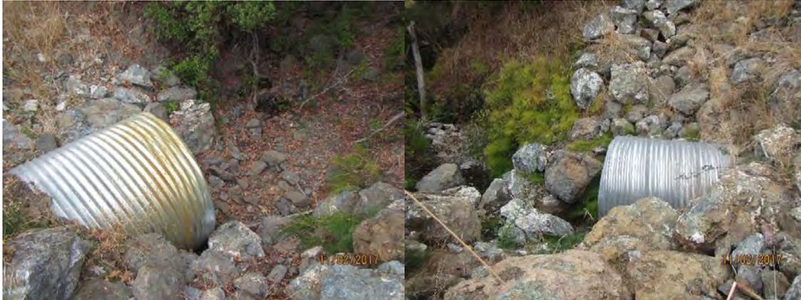
**Figure 13.** Substantial obstruction of the natural flow and alteration of the bed, bank, and channel of an unnamed tributary to Bear Creek and the South Fork Eel River by the placement of a culvert and fill within the channel.
