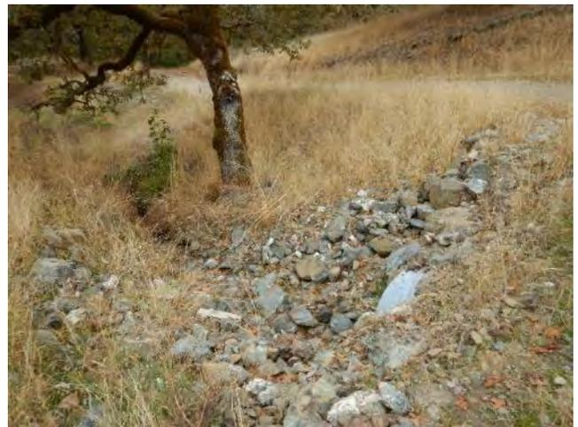
Photo 46: Image of downstream side of stream crossing C4 showing armoring of streambed and banks.
