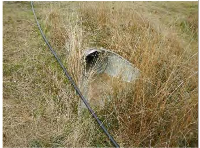
Photo 8: Closer view of POND1 outflow pipe (OUT1) with a layer of sediment covering the bottom of intake.
