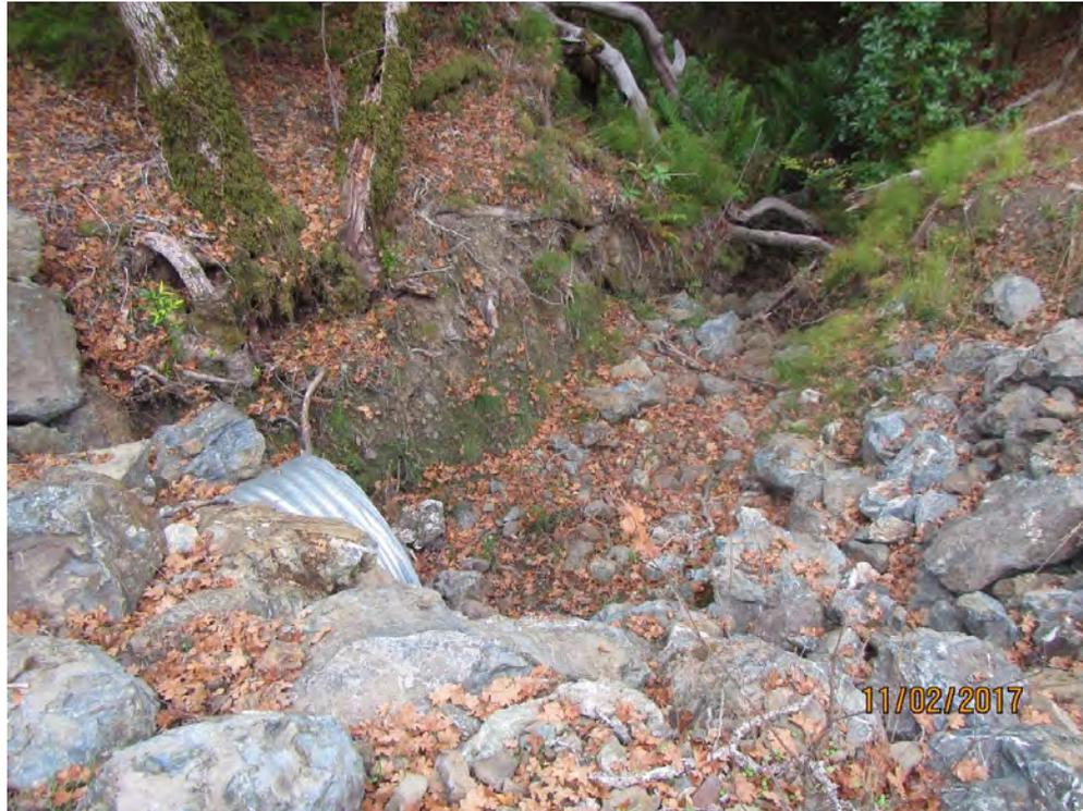
**Figure 7.** Substantial obstruction of the natural flow and alteration of the bed, bank, and channel of an unnamed tributary to Bear Creek and the South Fork Eel River by the placement of a culvert and fill within the channel.
