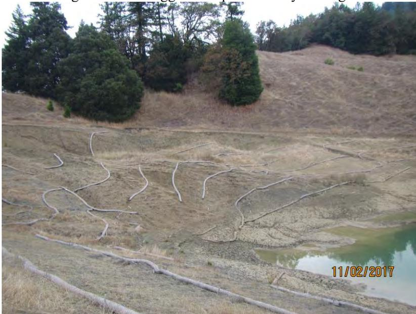
**Figure 5C.** Substantial discharge of sediment to Waters of the State from unpermitted grading and pond construction that removed vegetation and triggered slope instability leading to land sliding into the pond and then into the on stream pond.
