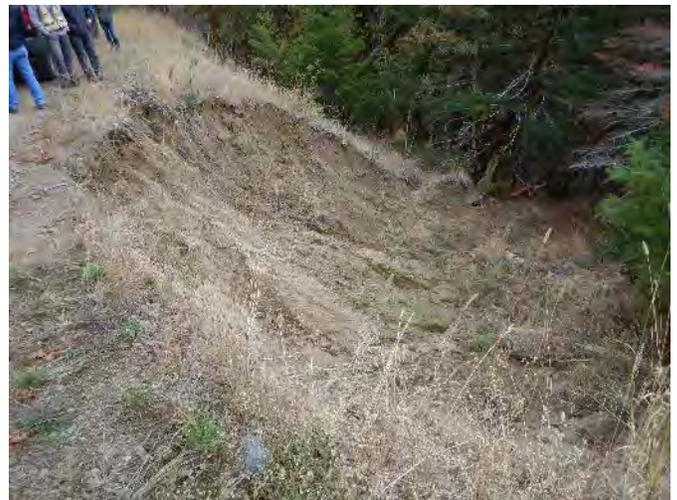
Photo 38: Image of landslide (SLIDE2) downgradient of the road located between stream crossing C2 and POND1 caused by road development, grading and surface runoff.
