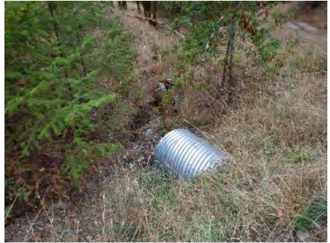
Photo 48: Image of downstream side of stream crossing C5 showing the culvert not set to the grade of the streambed.
