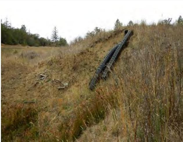
Photo 17: Image of double outflow pipes from POND2 into wetland type area (OUT2).
