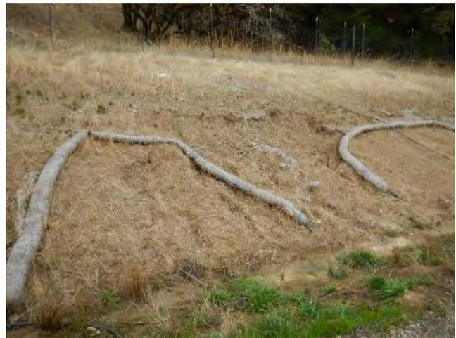
Photo 22: Image of drainage trench at outdoor cultivation area CA1. Image also shows fiber rolls disturbed by soil slumps caused by vegetation removal and erosion of the graded hillside. The fiber rolls were not functioning.
