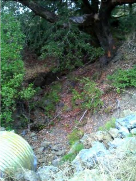
Photo 51: Image of upstream side of stream crossing C7 showing armoring of stream channel.
