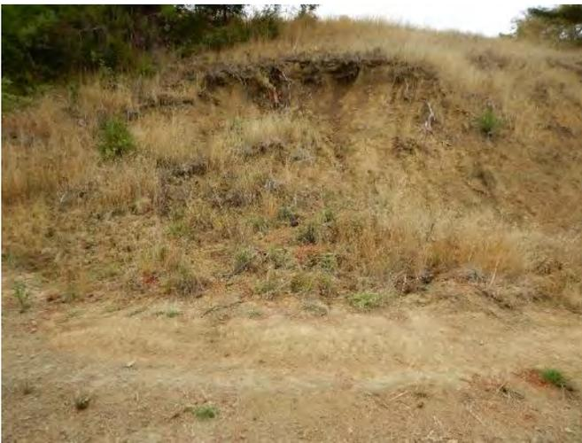
Photo 37: Image of landslide slope failure (SLIDE2) upgradient of the road, located between stream crossing C2 and POND1 caused by road development, grading and surface runoff.
