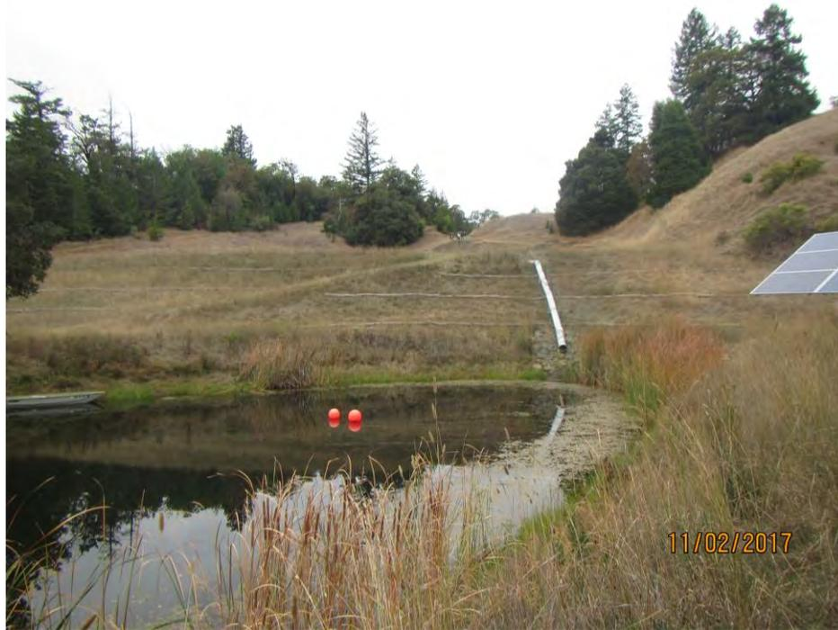
**Figure 5D.** Substantial discharge of sediment to Waters of the State from unpermitted grading and pond construction that removed vegetation and triggered slope instability leading to land sliding into the pond and then into the on stream pond.
