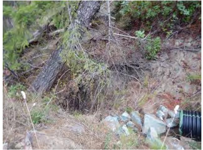
Photo 36: Image of downstream side of stream crossing C2 showing streambank erosion and stream bed armoring.
