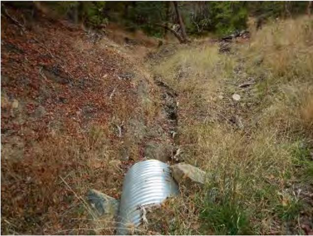
Photo 47: Image of upstream side of stream crossing C5 showing erosion of streambed.
