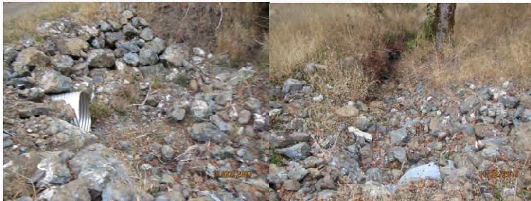
**Figure 8.** Substantial obstruction of the natural flow and alteration of the bed, bank, and channel of an unnamed tributary to Bear Creek and the South Fork Eel River by the placement of a culvert and fill within the channel.
