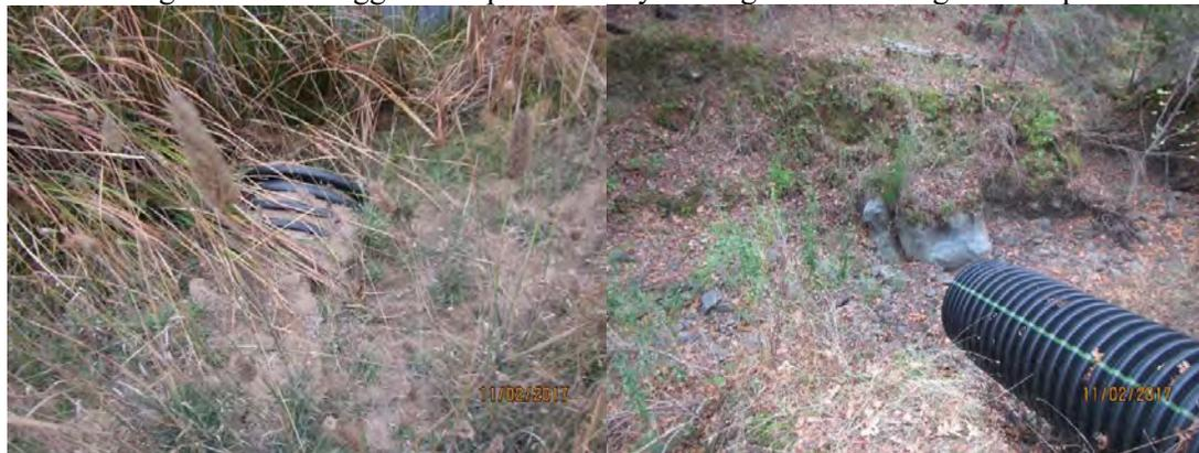
**Figure 6.** Substantial obstruction of the natural flow and alteration of the bed, bank, and channel of an unnamed tributary to Bear Creek and the South Fork Eel River by the placement of a culvert and fill within the channel.
