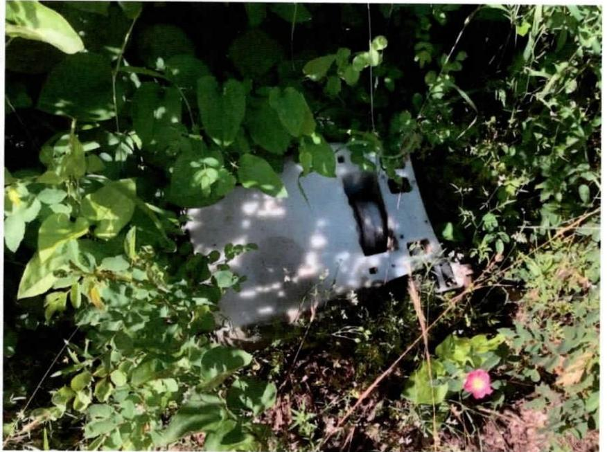
**Photo 26 and 27:** Water diversion and screened 1 ¼ inch intake at Water Source 1 (WS-1) on Chapman Gulch.
