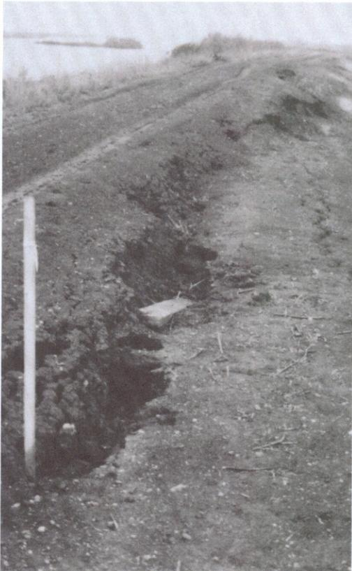
*Cracks occurring on the levees of a low-lying island.*
