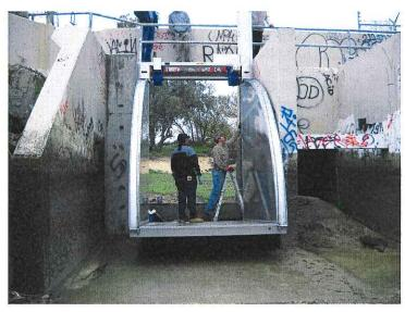
Above: Downstream view of the open flume gate during installation
