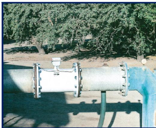
*Figure 3-16. Magnetic Flow Meter*
