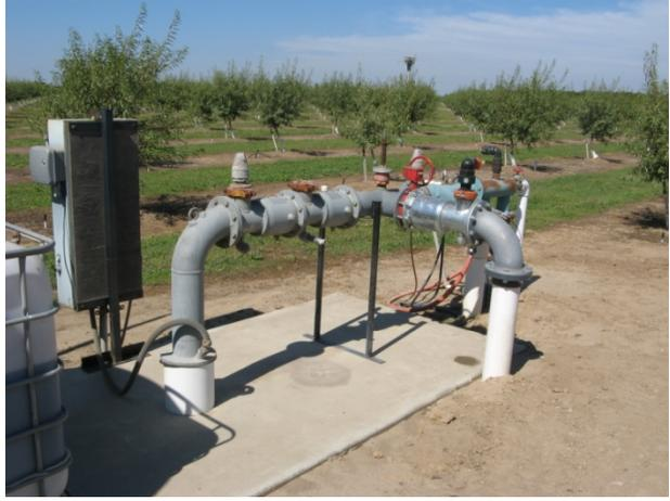
**New Solid Set Sprinkler System and Division 9 Dual Groundwater Surface Water Turnout.**
