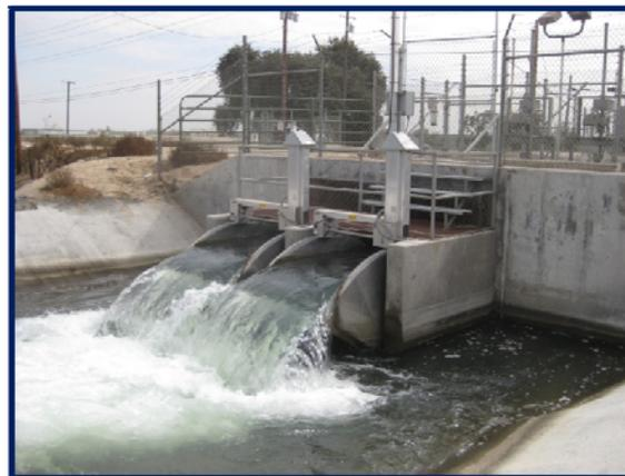
*Figure 3-5. Flume Gates at Lateral Heading*
