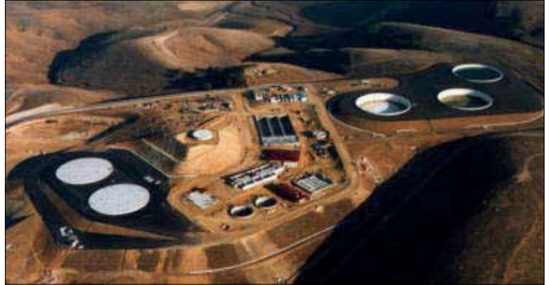
Polonio Pass Water Treatment Plant
