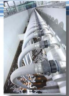
Microfiltration (MF) is a separation process that uses polypropylene hollow fibers, similar to straws, with tiny holes in the sides that are 0.2 micron in diameter (1/300 the diameter of a human hair). By drawing water through the holes into the center of the fibers, suspended solids, protozoa, bacteria and some viruses are filtered out of the water.
